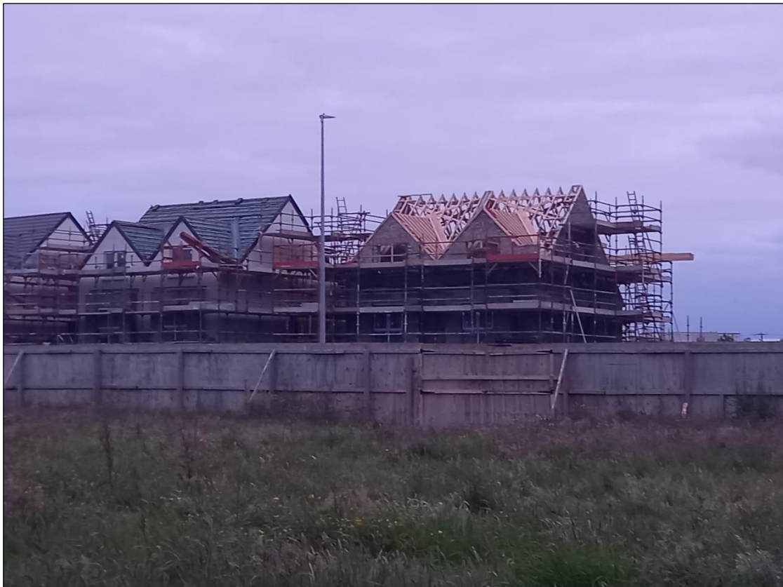
Plate 5-4 Hoarding present along the southern boundary of the proposed development site.
