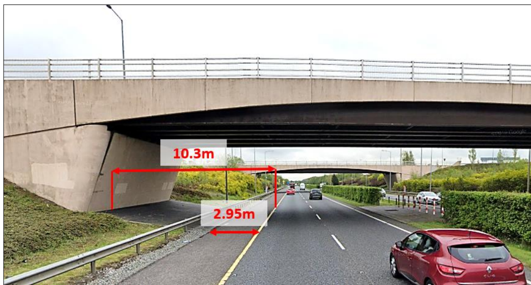
Figure 3.8: Junction 6 Overbridges (West Bridge) (©2021 Google)
