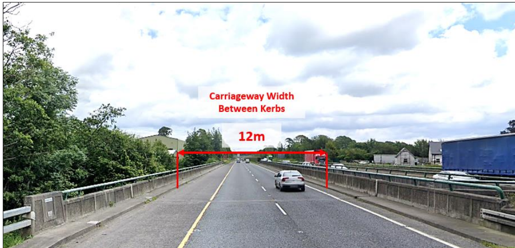
Figure 3.10: Liffey River Bridge – (©2021 Google)
