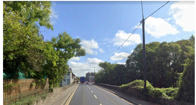
Fig 36. View eastward over bridge to town entry point
