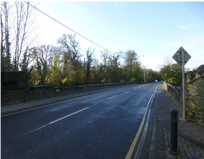
Fig 27. View west over bridge - upper section of bridge structure is in relatively good condition
