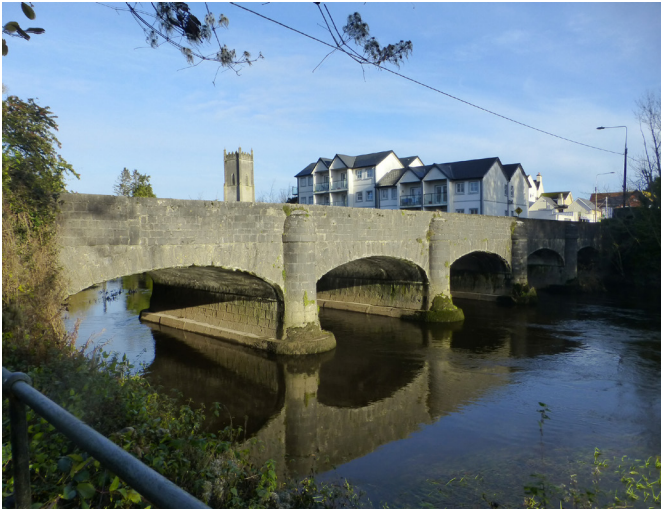
Fig 14. Southern side of bridge - downstream
