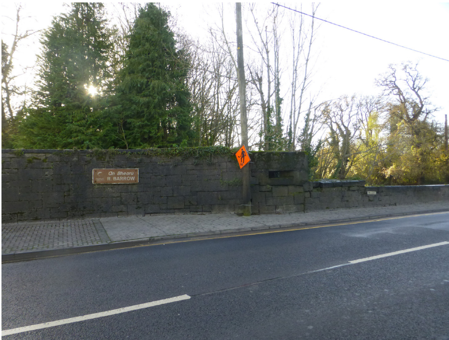
Fig 20. Concrete Pillbox integrated into the bridge parapet during the Emergency of 1939-45
