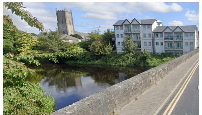
Fig 37. View to east bank to north side of bridge
