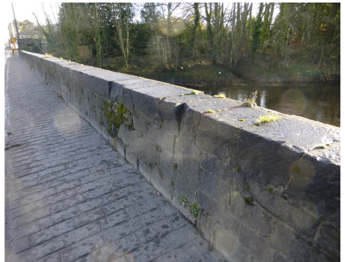
Fig 28. Localised vegetation removal and pointing of open joints to parapet wall
