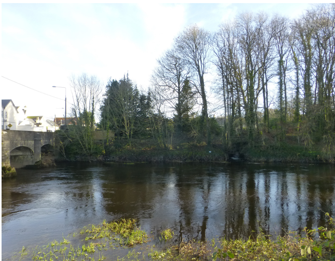
Fig 31. View to eastern embankment on downstream side of river. Scouring has been identified along river edge and rock armour protection is proposed along river
