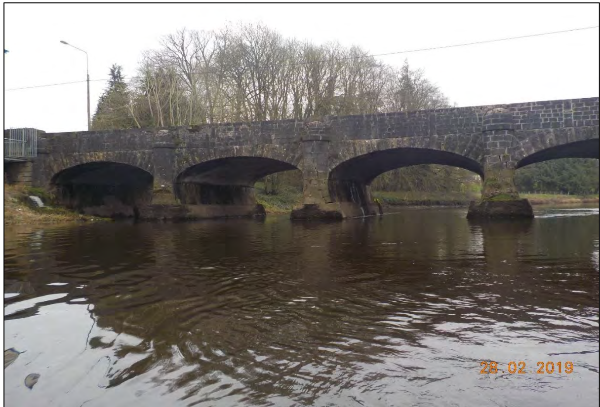
Figure 1: Monasterevin Bridge Upstream Elevation
