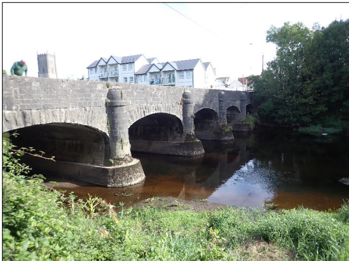
Plate 1 Monasterevin bridge viewed from downstream.
