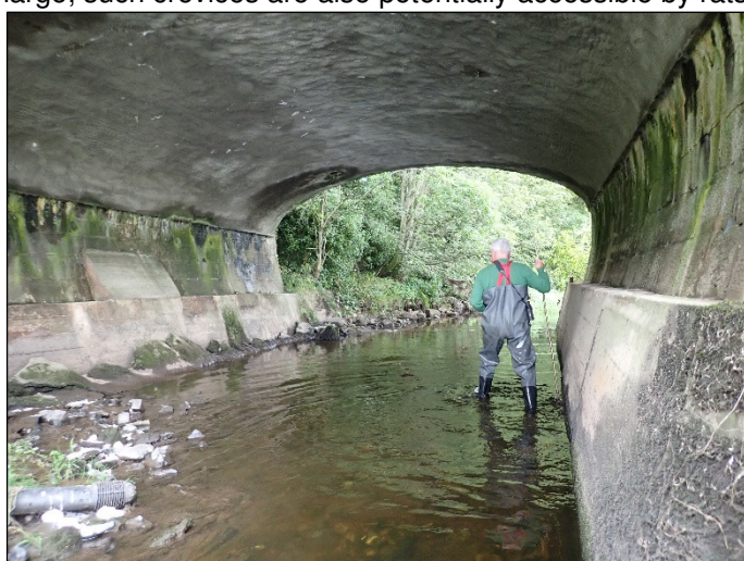
Plate 12 Left arch also showing previous filling / repointing. Only crevices at the top of the bridge are wet and seem to be receiving road runoff – making them unsuitable for use by bats.
