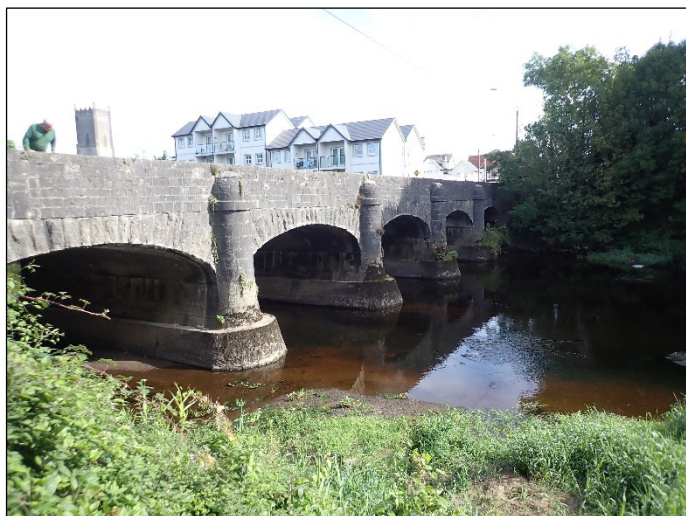
Plate 1 Monasterevin bridge viewed from downstream.
