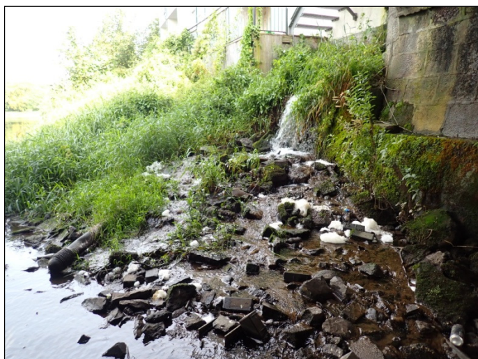
Plate 8 Sewage inlet flowing over litter and debris into the Barrow channel on the upstream left bank.
