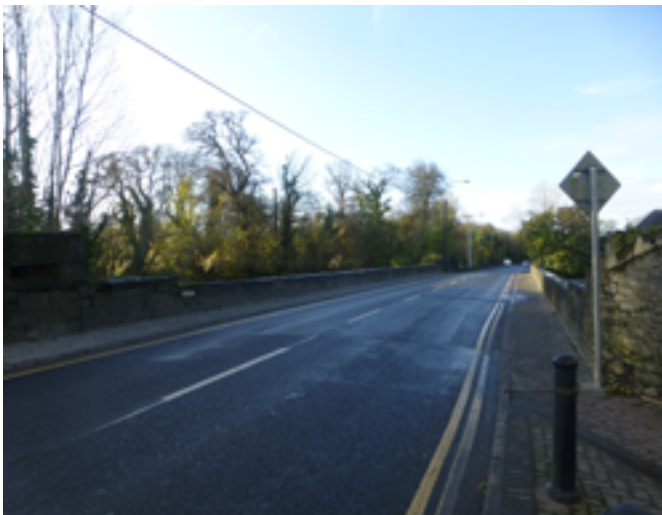
Fig 27. View west over bridge - upper section of bridge structure is in relatively good condition
