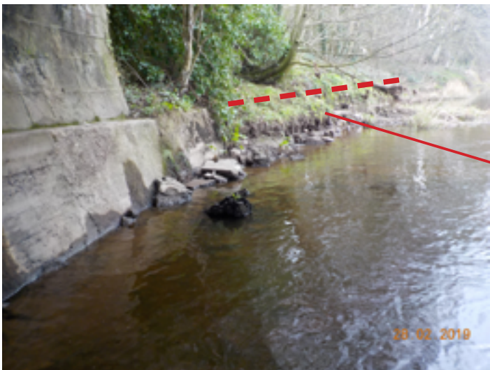
Fig 33. Scouring erosion along east embankment. Rock armour protection proposed to edge
