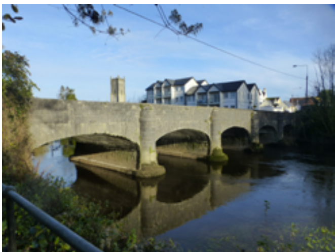
Fig 22. Impressive 5-span elliptical arched bridge spanning the River Barrow
