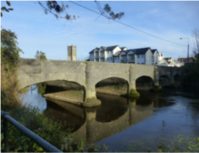
Fig 14. Southern side of bridge - downstream
