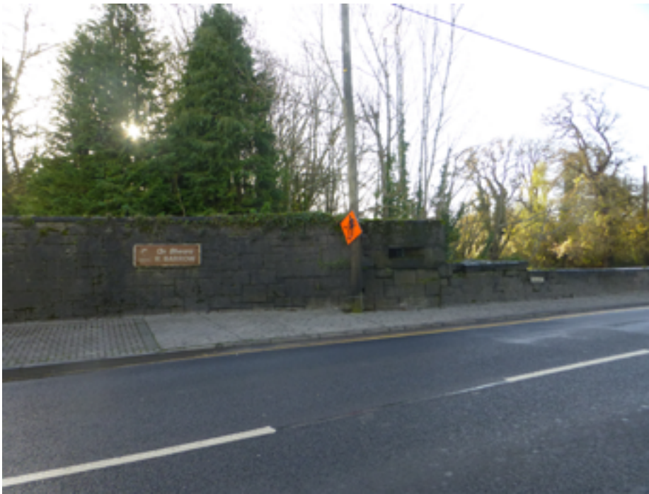
Fig 20. Concrete Pillbox integrated into the bridge parapet during the Emergency of 1939-45
