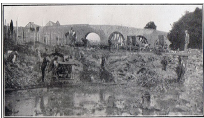
Plate 11 Dredging works at Monasterevin in the 1930s. This entire stretch of river was dredged and channelised and the effects of this scheme are still apparent today (Source: Irish Waterways History).
