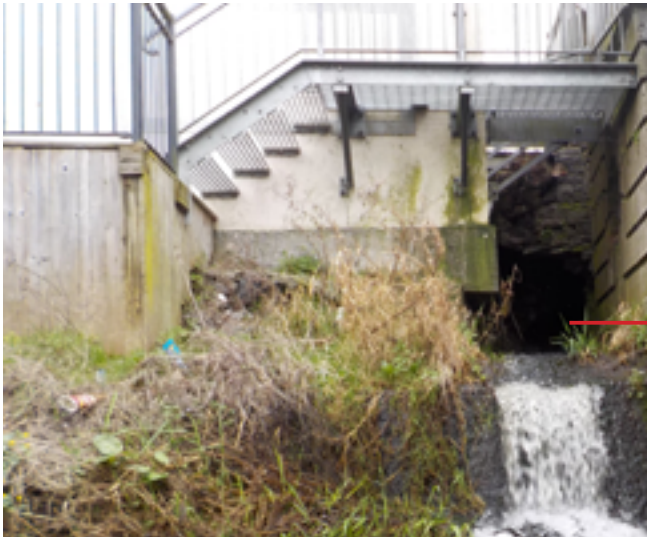
Fig 32. Outfall from original mill pond that served the distillery on the east embankment
