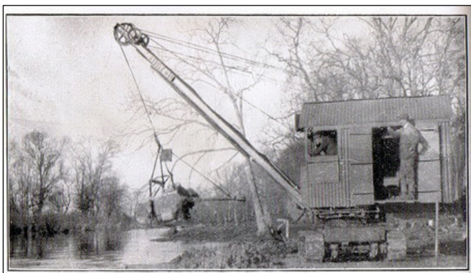
Plate 6 Dredging works at Monasterevin in the 1930s. The dredging works were undertaken using drag lines and the river was also diverted and dried out during the works. This scheme permanently altered the physical character the river (Source: Irish Waterways History).
