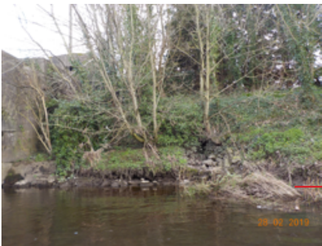
Fig 34. Masonry wall on east embankment will require rebuilding once trees are removed. Partial collapse has occurred. Wall may align with a structures built to infill water body indicated on the 1837 OS map in the later part of the nineteenth century
