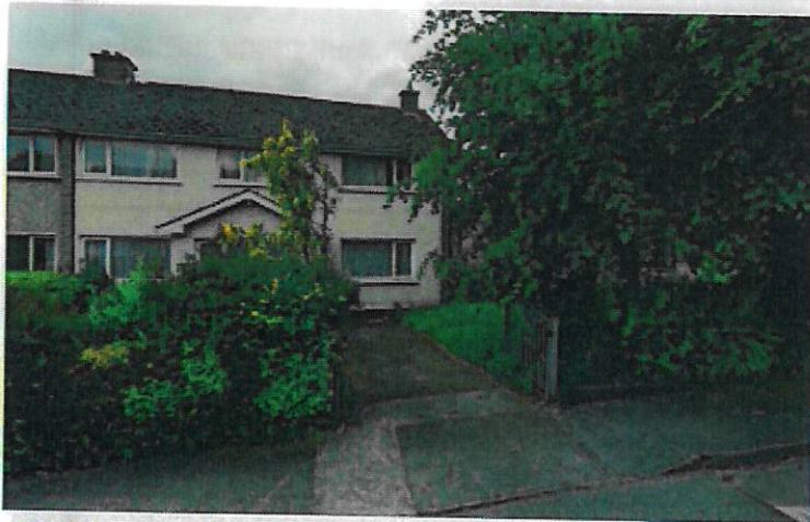
IMAGE 1. VIEW FROM PATRICIAN AVENUE-FRONT OF EXISTING HOUSE
