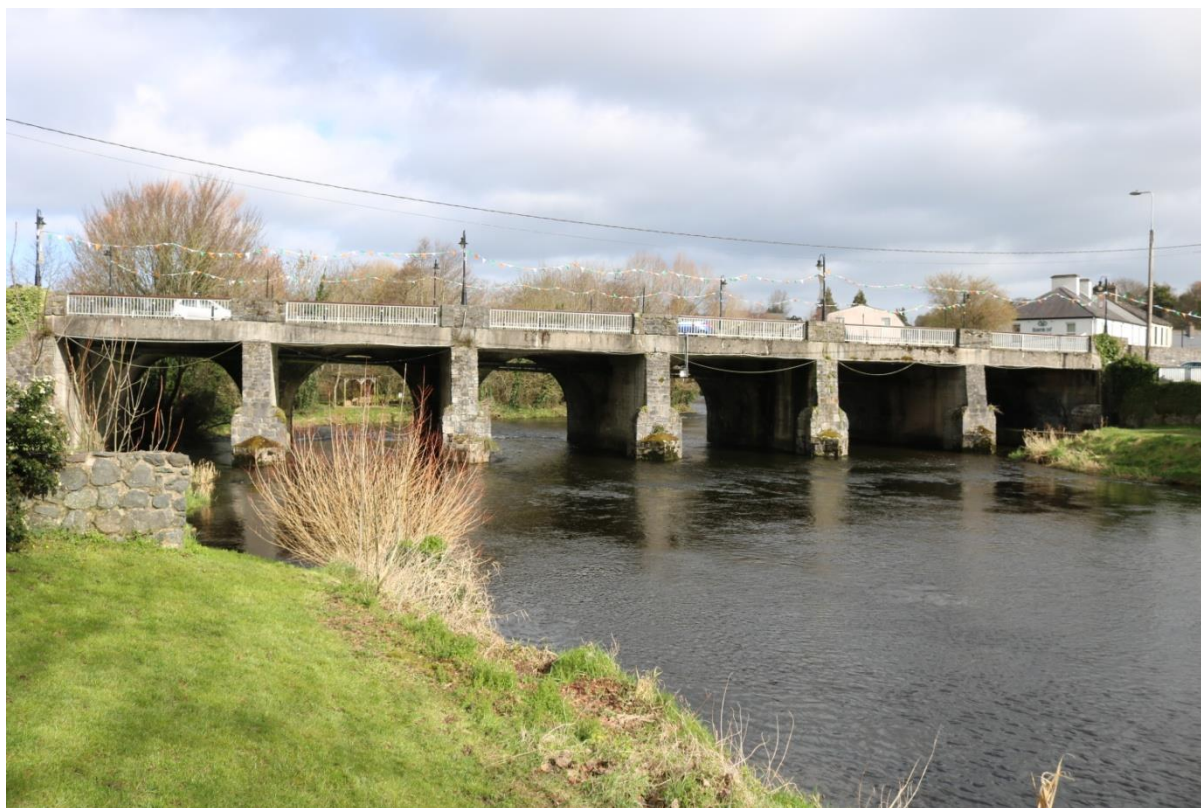
Figure 15: Kilcullen Bridge, from south, with c. 1970 widening of carriageway
