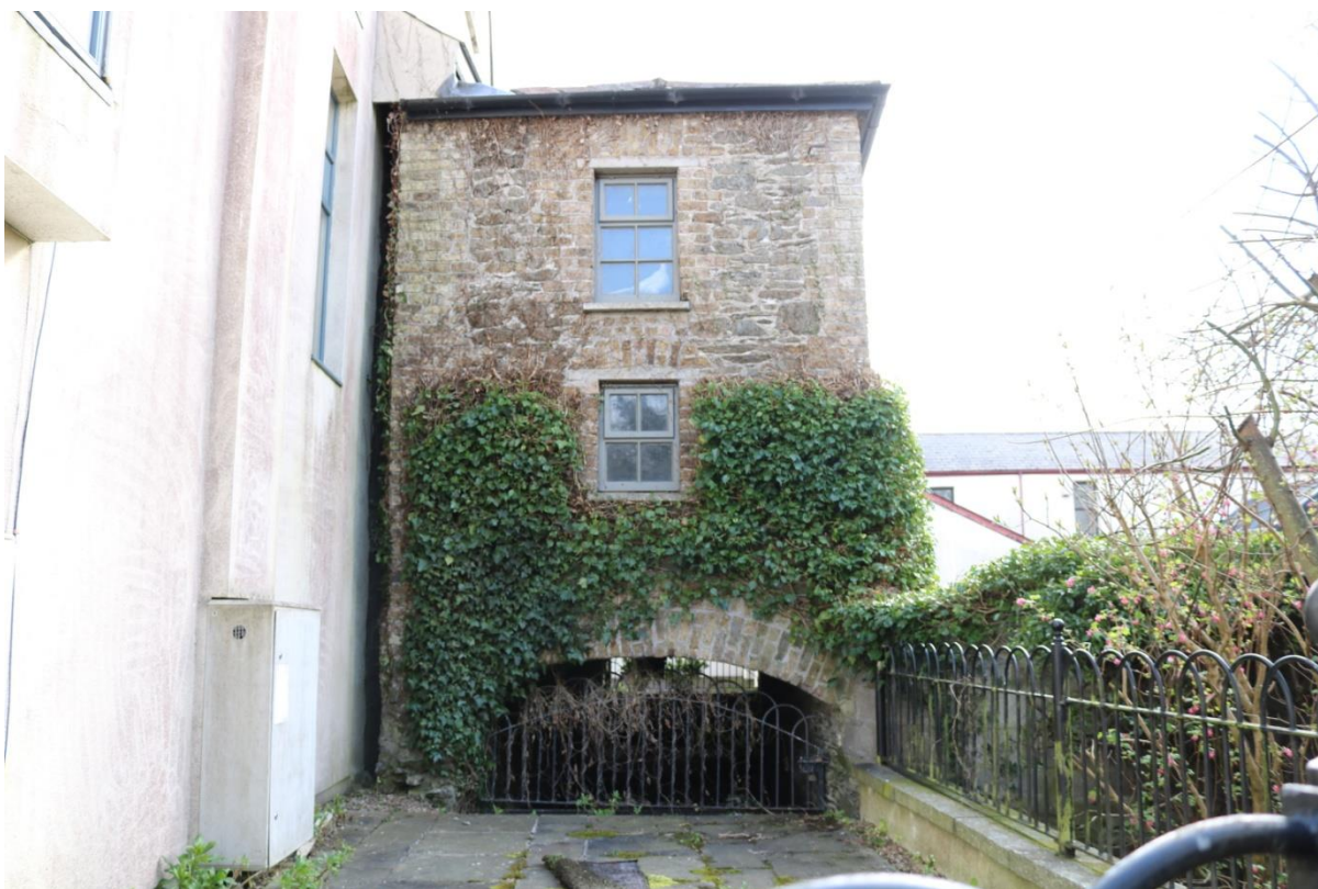
Figure 17: Part of former Corn Mill, from west
