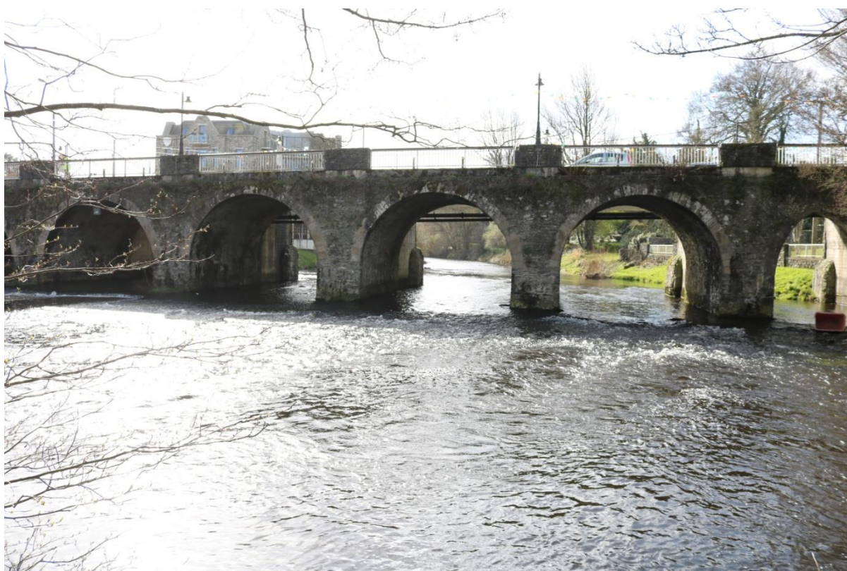
Figure 14: Kilcullen Bridge, from north
