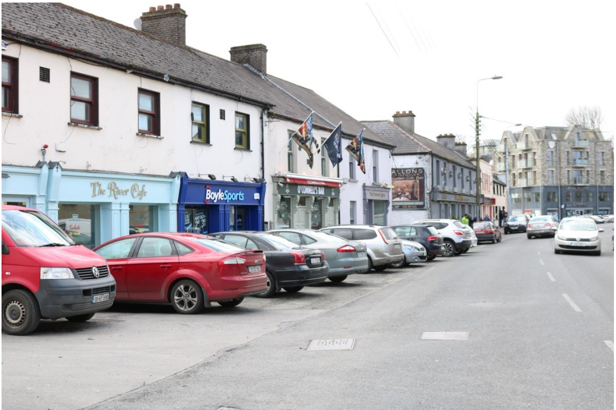
Figure 20: Lower Main Street, west side, from east
