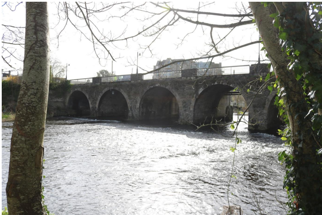
Figure 4: Kilcullen Bridge, from north
