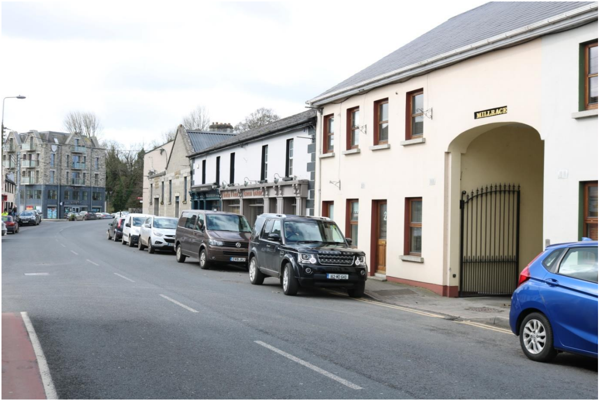
Figure 19: Lower Main Street, north side from east
