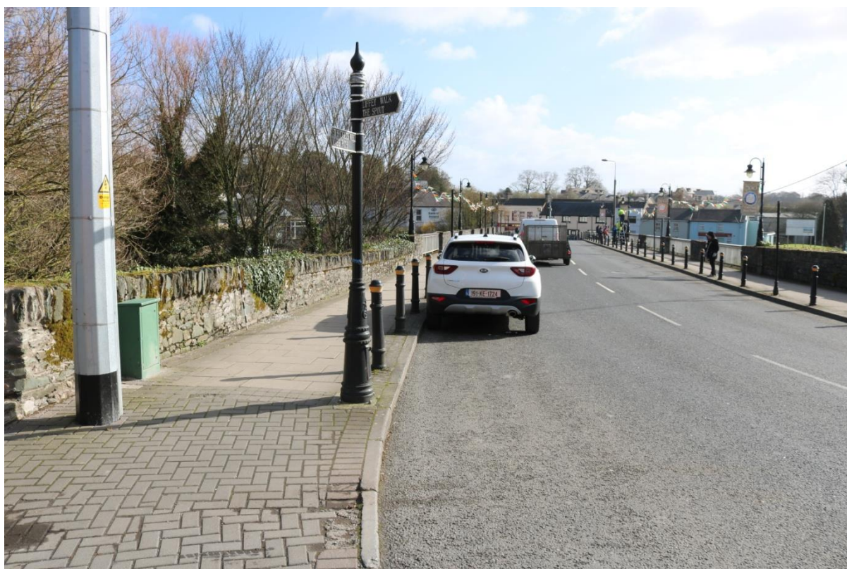
Figure 13: Kilcullen Bridge from west
