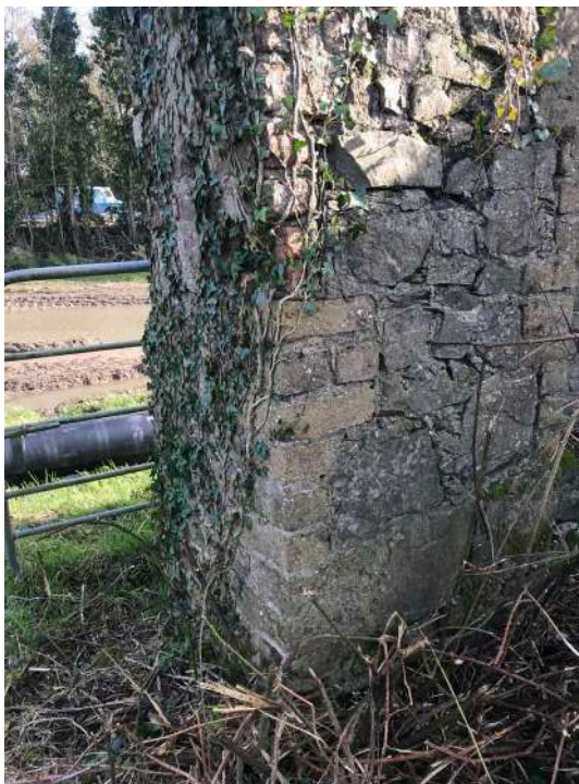
Edge of original doorway evident
