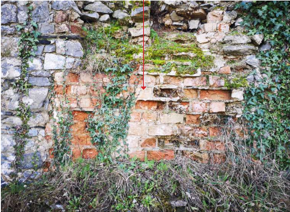
Detail at inside of southern wall
