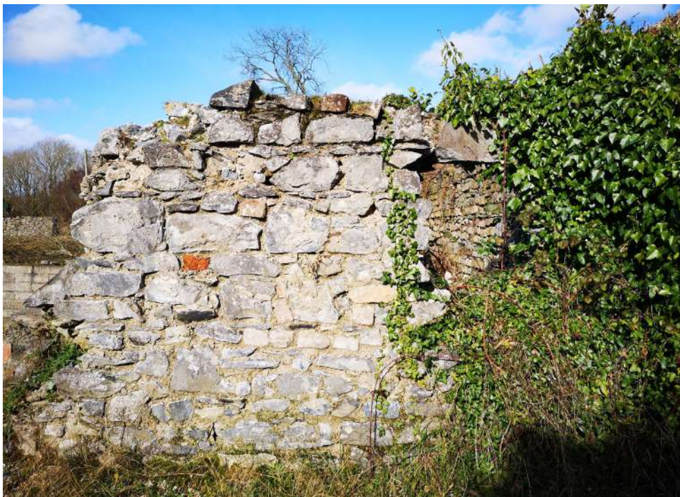
Evidence of early window opening with stone lintel
