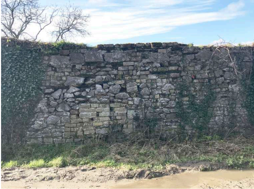
View of eastern courtyard wall
