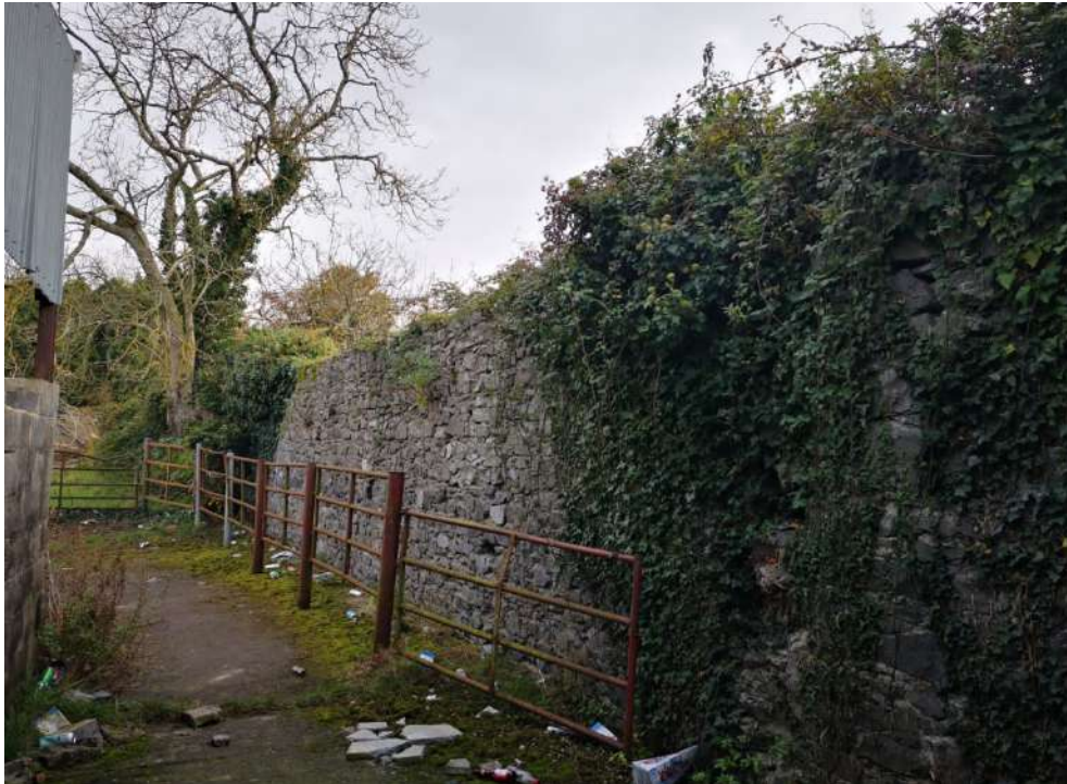
Substantial rubble stone wall to south boundary of rear courtyard
