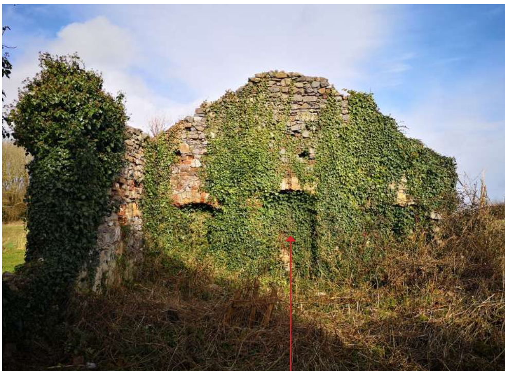
View of Northern gable with 3 no. blocked bricked arched openings
