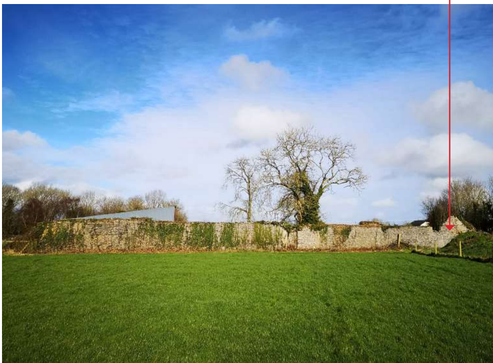
View of substantial stone wall to rear farm courtyard
