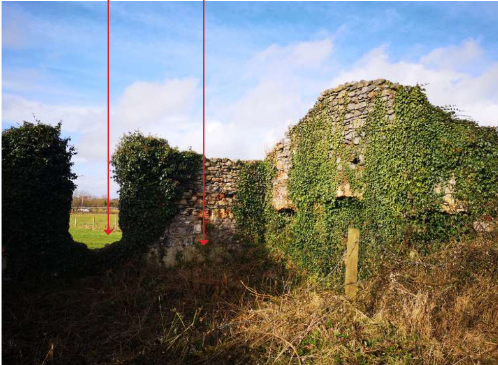
View of inside of north-west ruin
