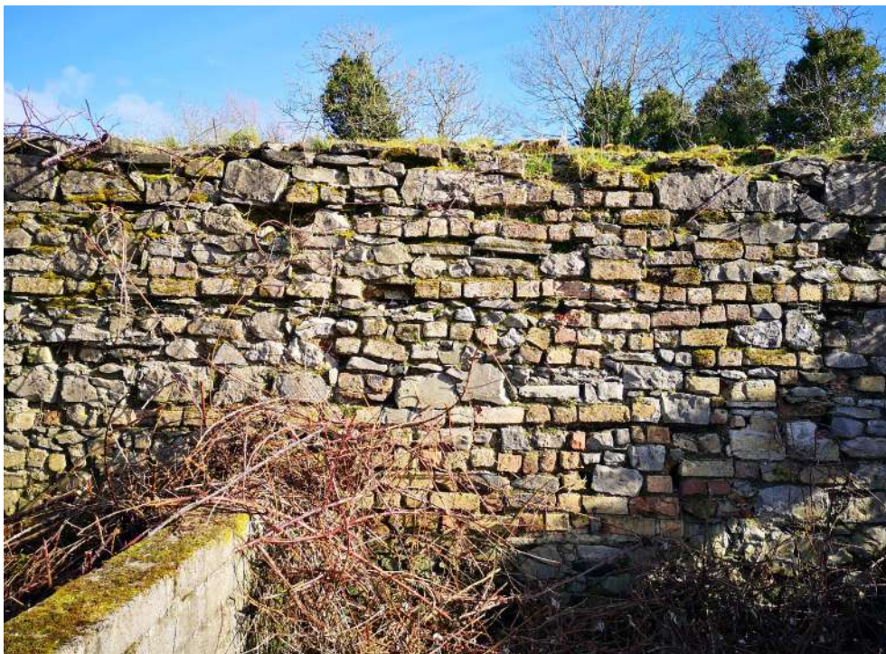
Detail of coursed brickwork to eastern wall of rear courtyard
