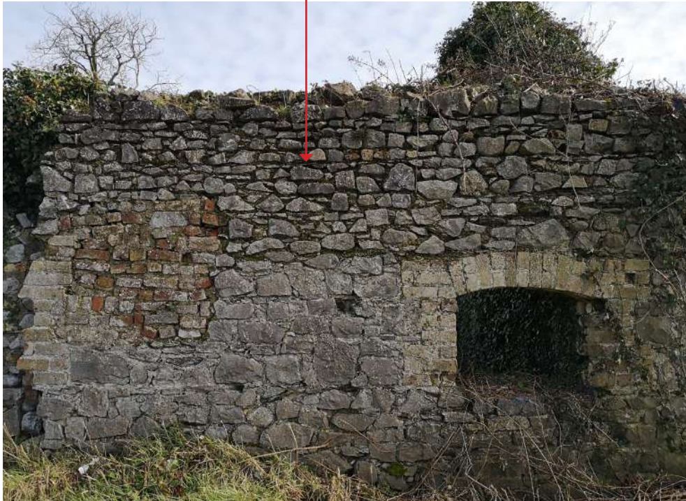
Detail of original building fabric of western ruin
