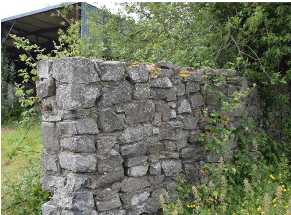
Detail of stonework to courtyard wall
