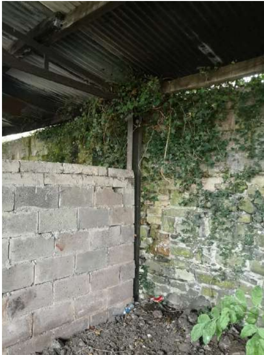
Concrete blockwork wall perpendicular to stone wall to West
