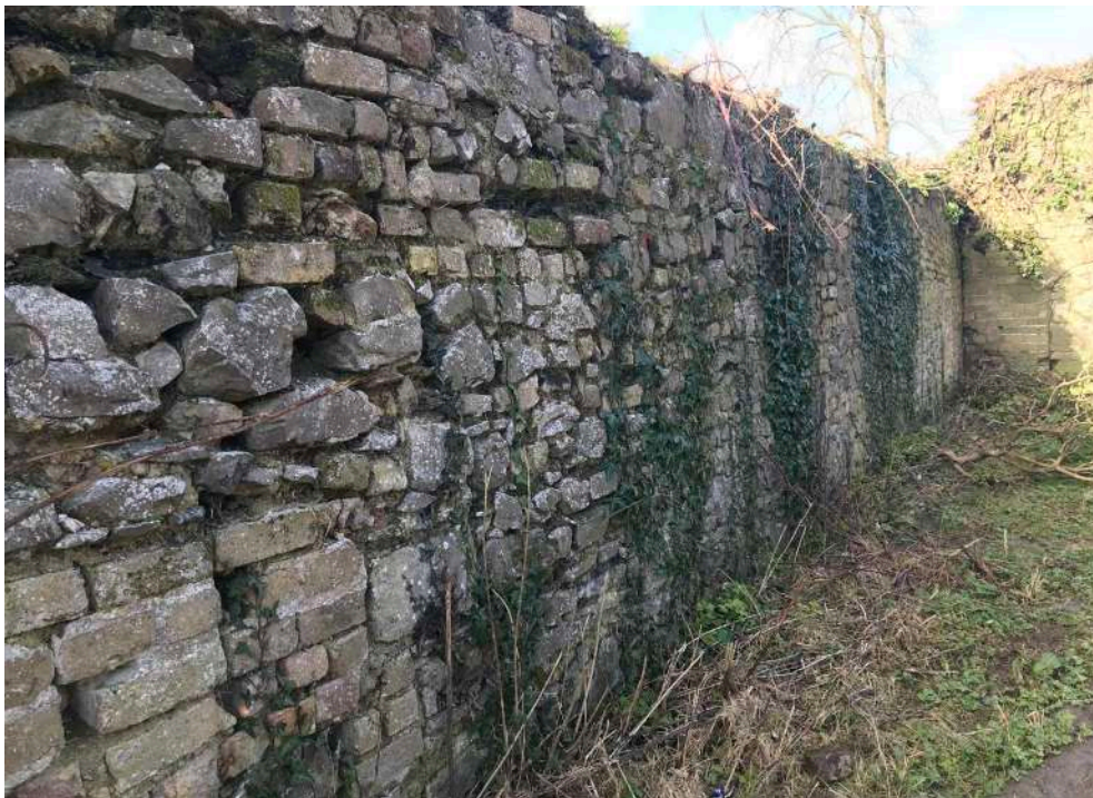
Detail of brickwork and stone to eastern courtyard wall
