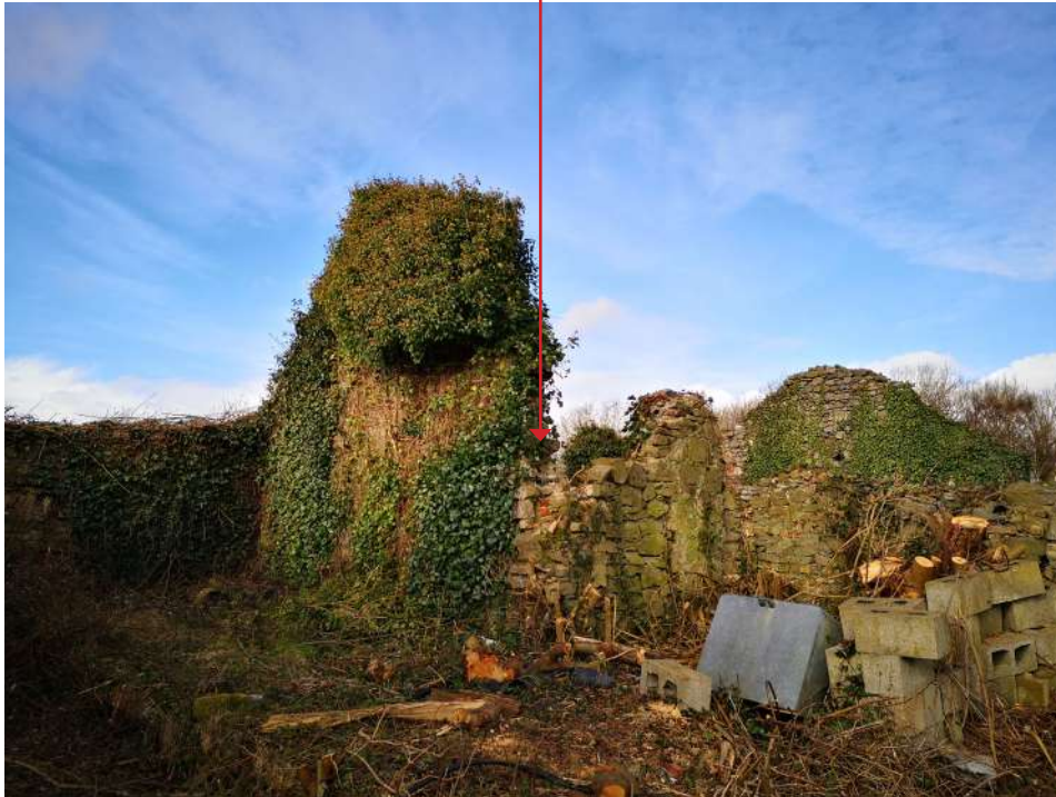
View of southern gable of North-West ruin
