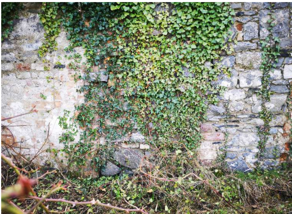
View of blocked arched opening to base of gable
