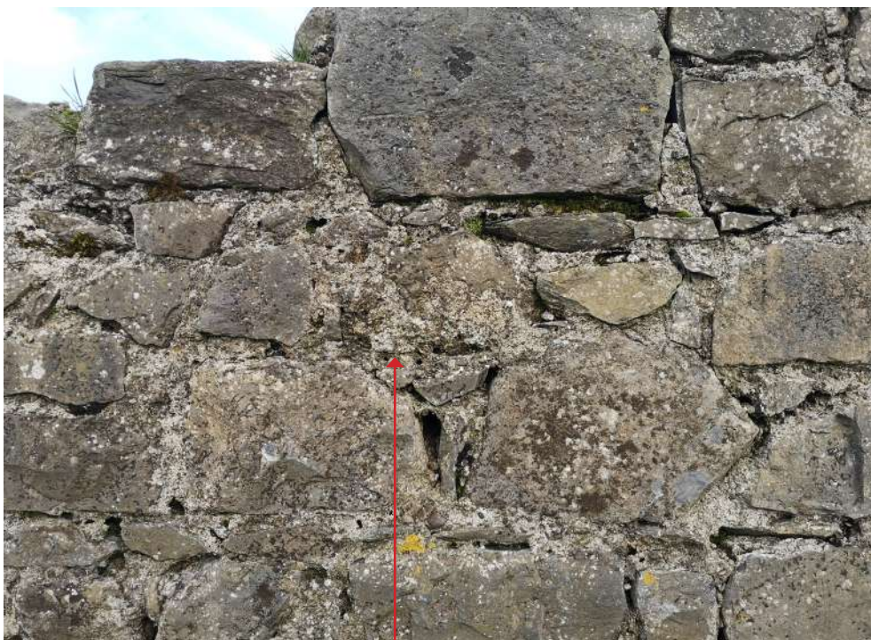
Lime mortar pointing evident to original exposed stonework
