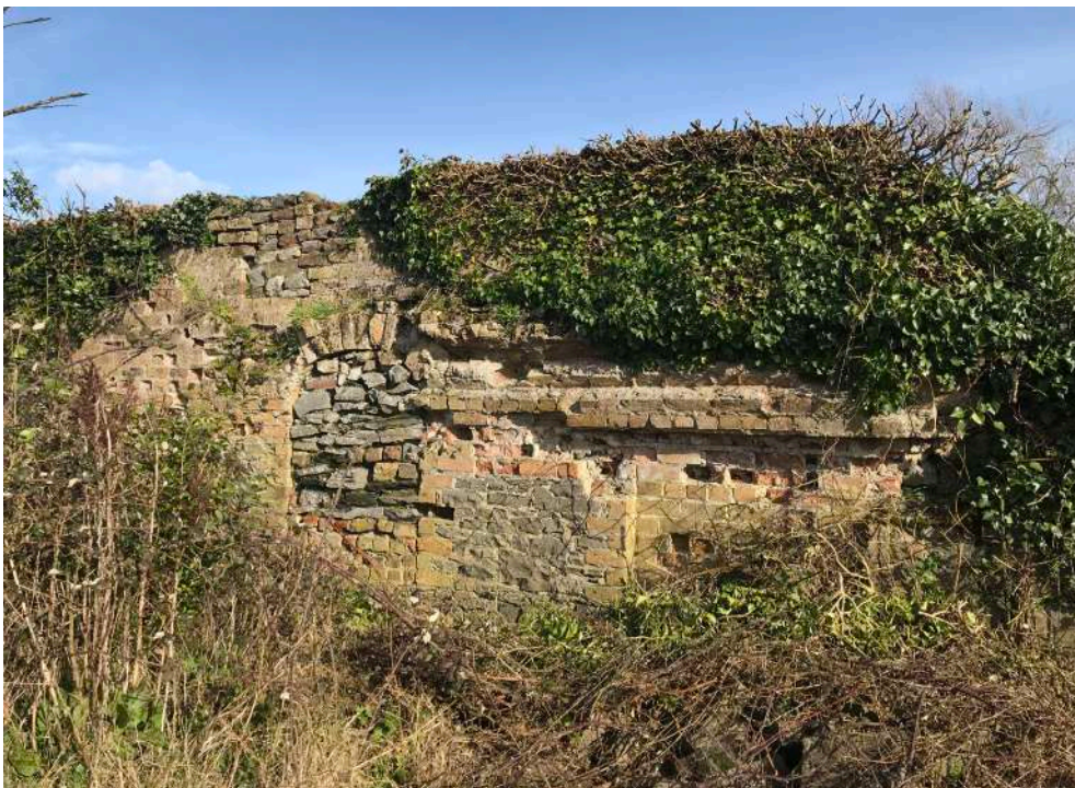
Brickwork coursing evident to Eastern wall of ruin
