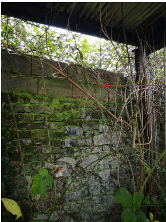
Concrete blockwork wall on stonewall to West
