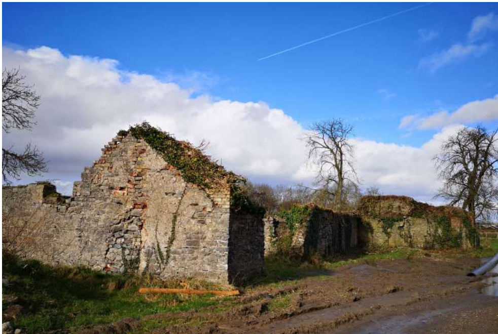
View of South-Eastern ruin and Eastern ruin beyond
