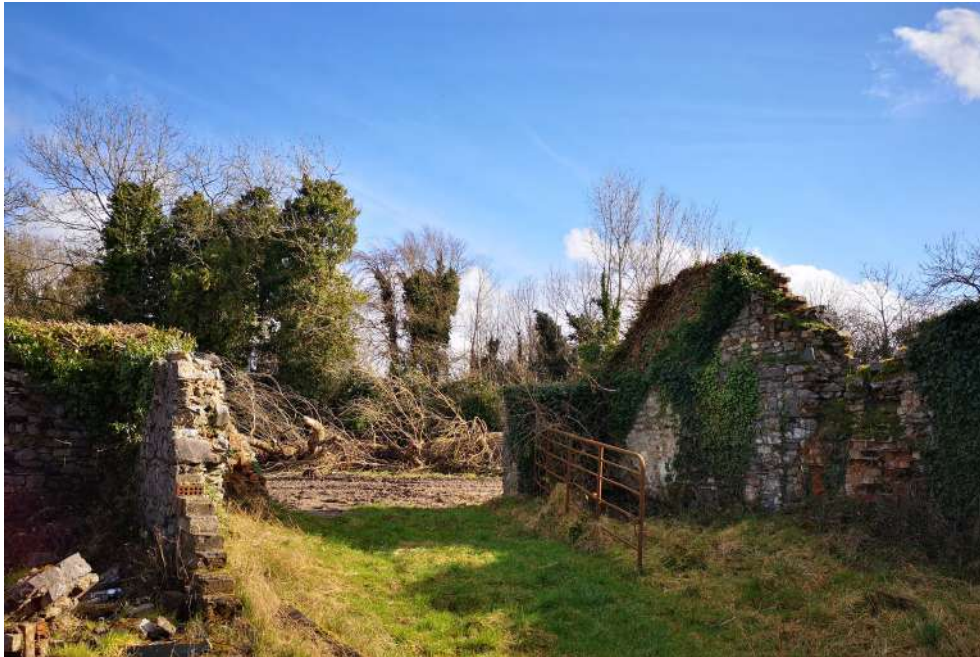
View inside remains of South-Eastern ruin
