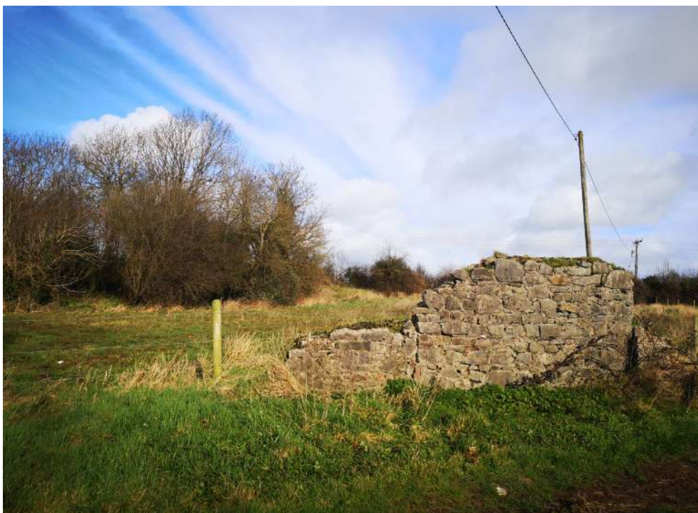
Exposed stone work to original farmhouse
