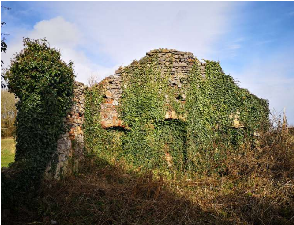
View of remains of northern gable with blocked brick archways
