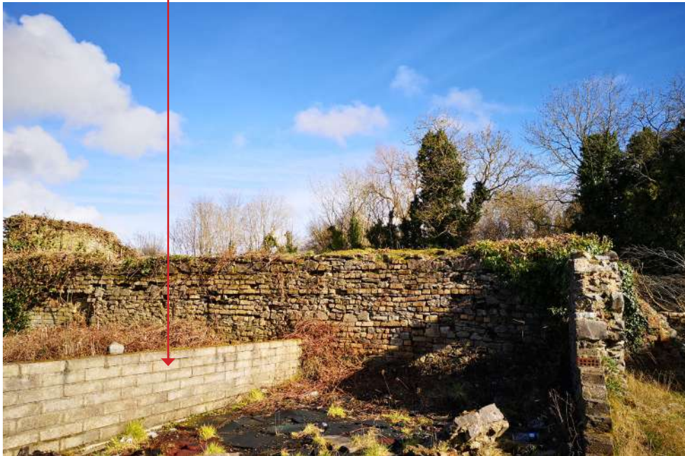
View of brickwork wall to eastern side of courtyard
