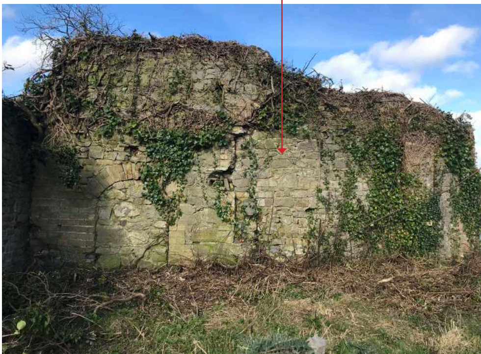
View of low arched opening to gable wall
