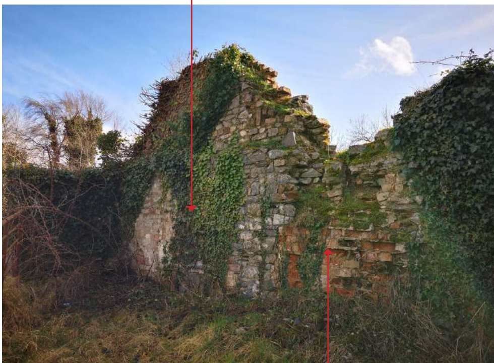
Surviving Southern Gable of South-Eastern Ruin
