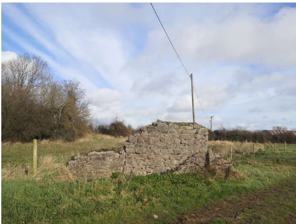
View of exposed stone work to remains of farmhouse
