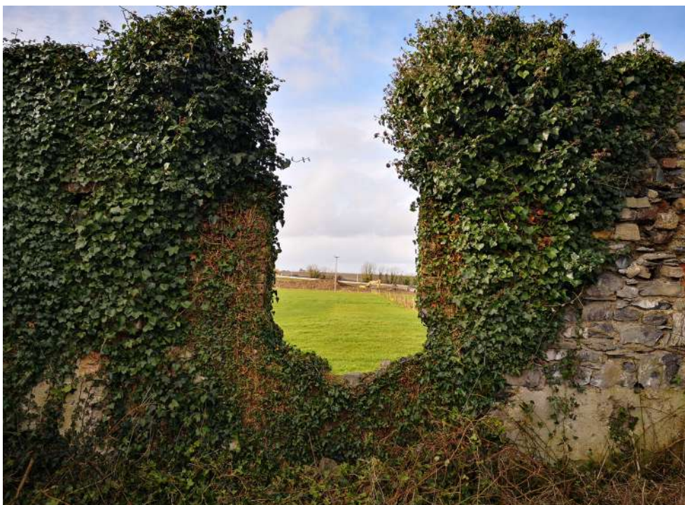
View of rear courtyard and ruined outbuildings to the Eastern boundary
