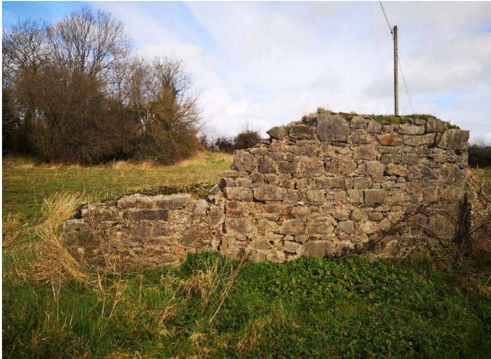
No original lime render evident to exposed stonework
