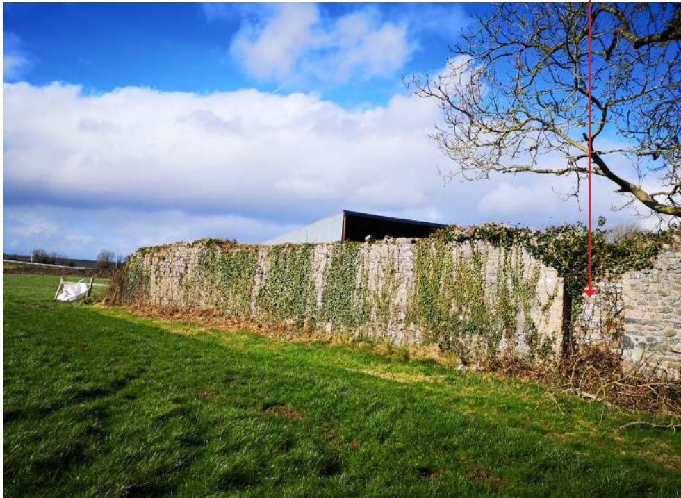
View of southern courtyard wall
