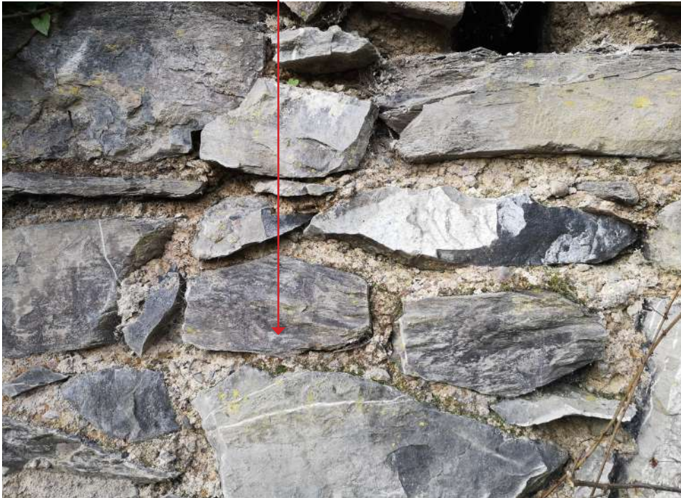
Detail of limestone exposed wall
