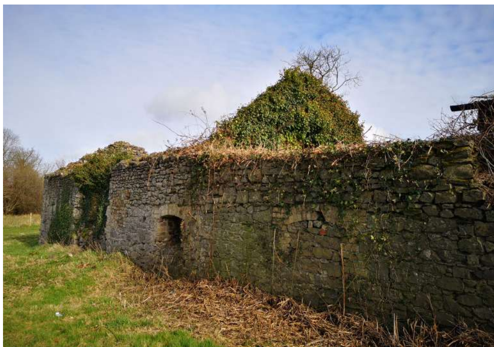
View of western ruin and arched openings
