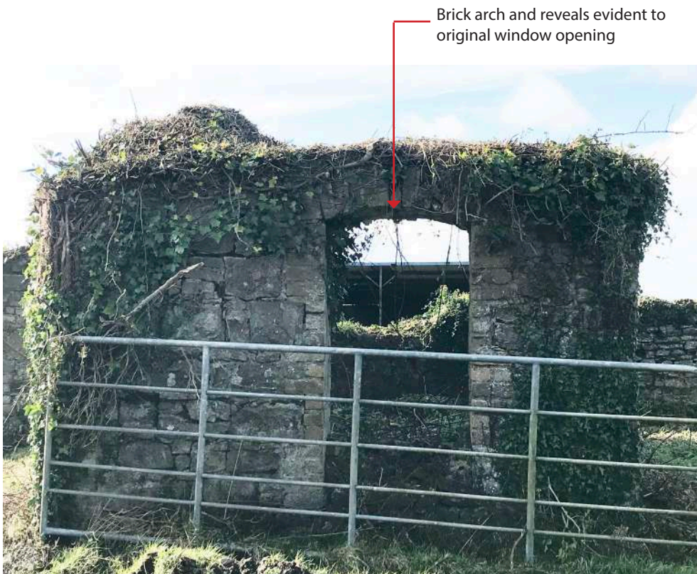
View from east of remains of eastern wall
