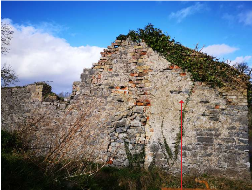
Limestone and brick fabric evident to Southern wall
