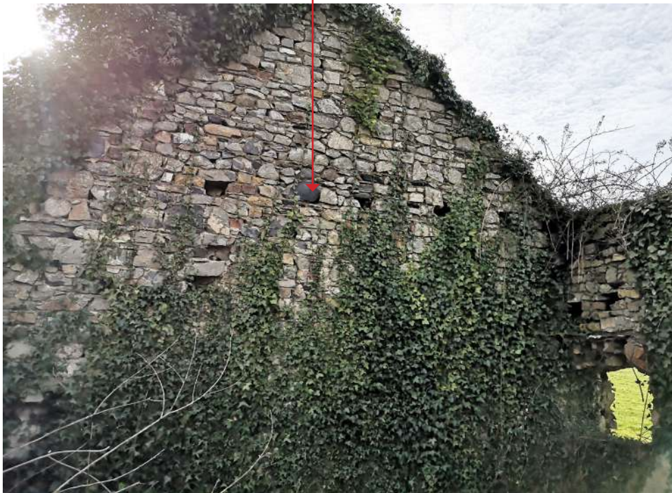
Southern gable wall of North-West Ruin
