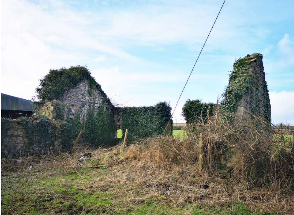
View of North-West ruin
