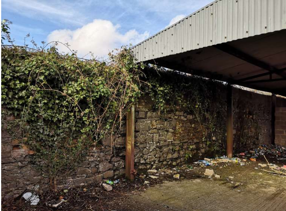
View of existing agricultural shed structure and steel supports to same to Western boundary
