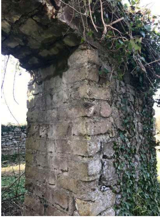
Detail of brick reveal to window arch
