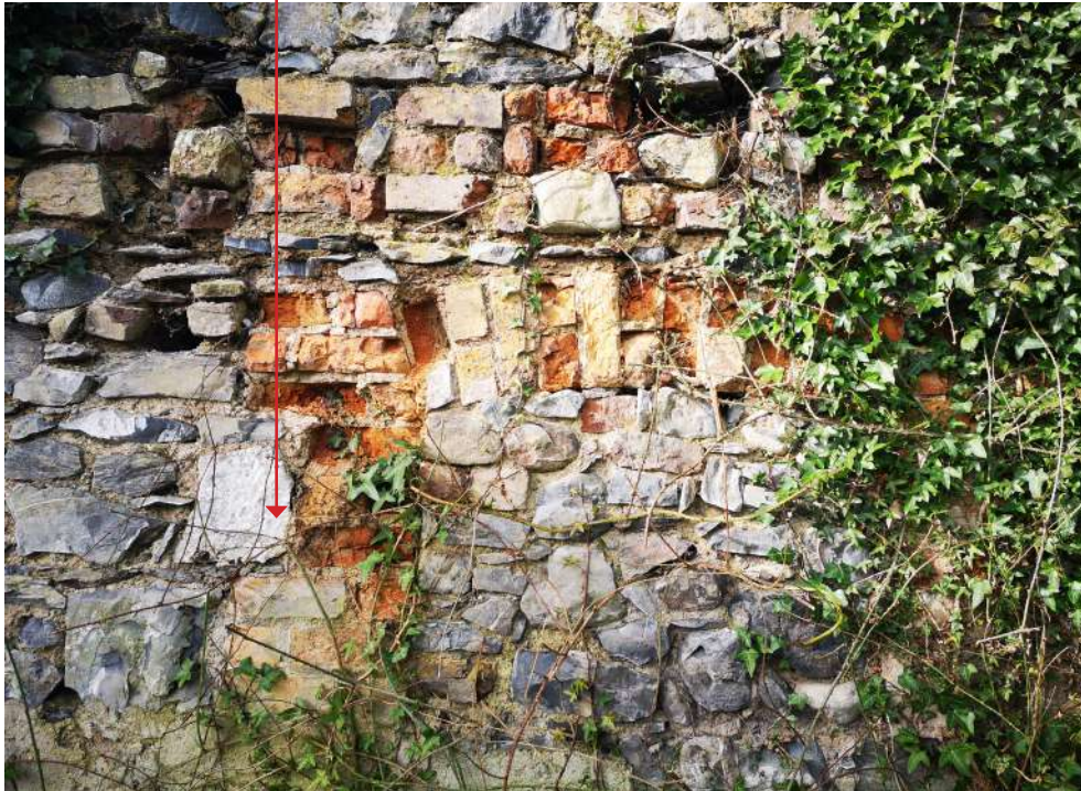
Detail of blocked brick arch
