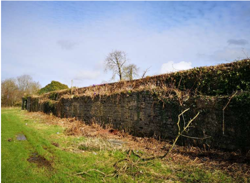
View of blocked arched windows to western ruin
