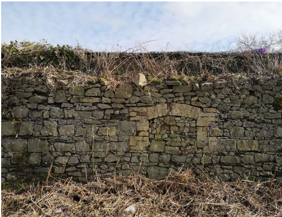
Detail of blocked arched window
