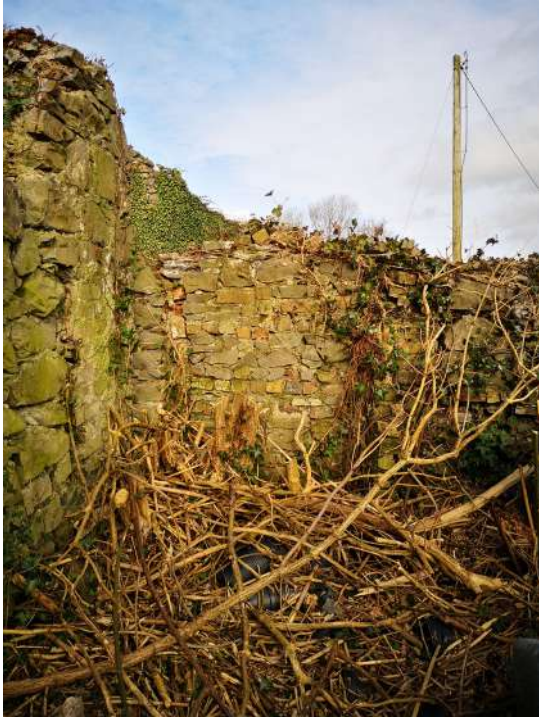
View of blocked opening to courtyard wall
