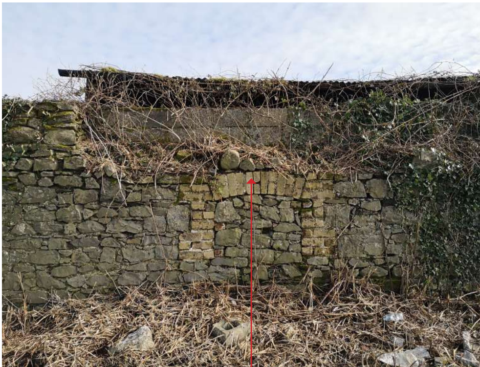
View of shallow brick arches evident along western wall
