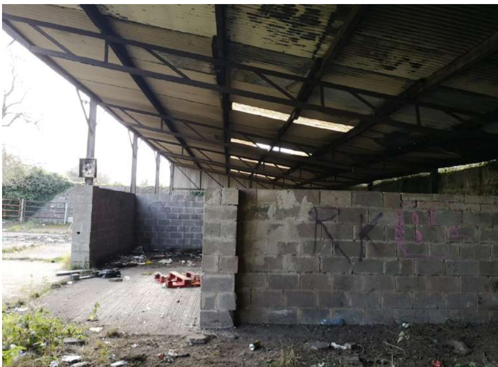
Mono-pitch roof to agricultural shed structure
