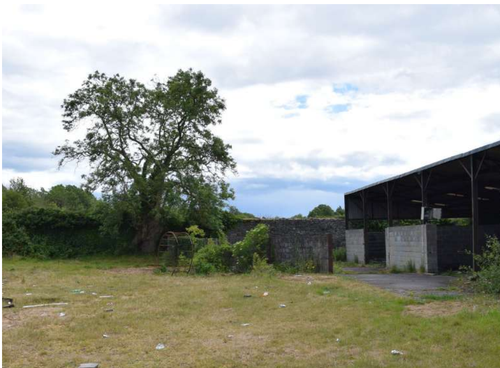
View within original rear 'working' courtyard looking south
