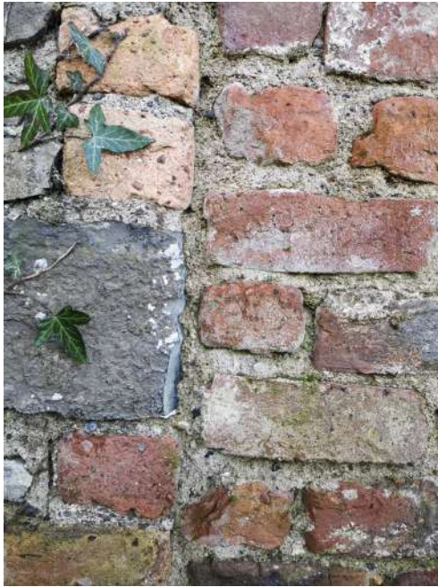
Detail of reveal to bricked arched door
