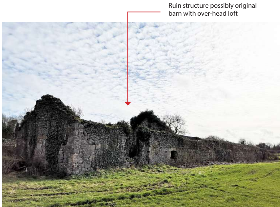
Substantial outbuilding to north-west
