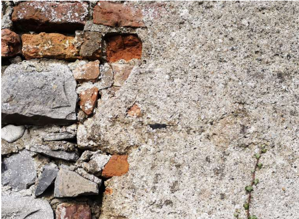
Detail of original wall fabric and lime render
