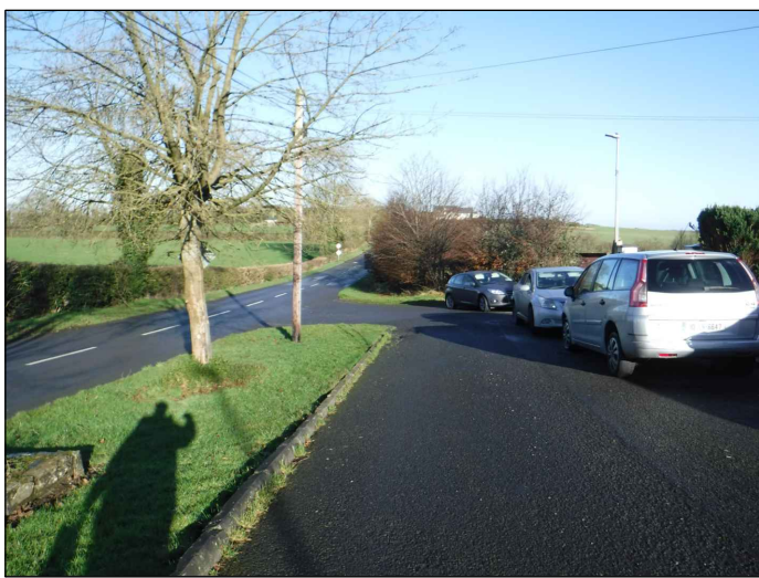
Calverstown Road View North along Access Road
