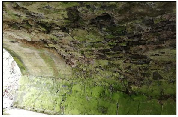
Figure 4: Crack in abutment and Arch Barrel
