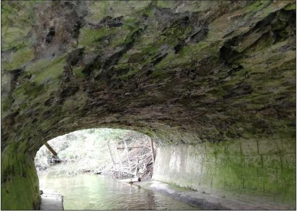
Figure 3: Loss of mortar in joints and vegetation growth
