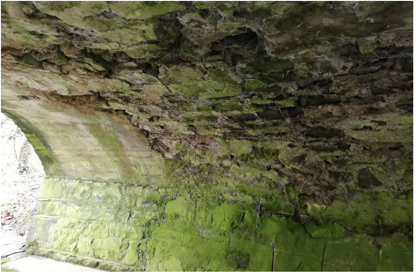
Plate 4: Crack in abutment and Arch Barrel
