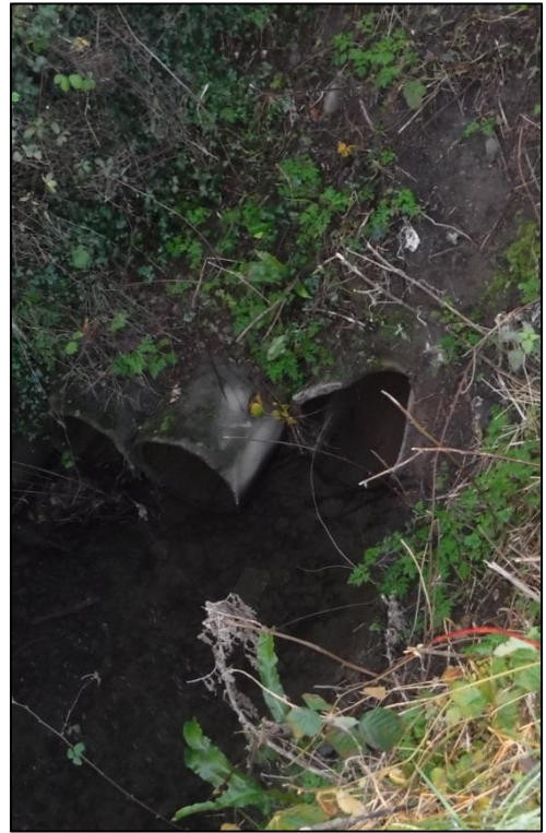
Plate 3 Concrete Pipes/Culvert to stream under R445 Road [VP2]
