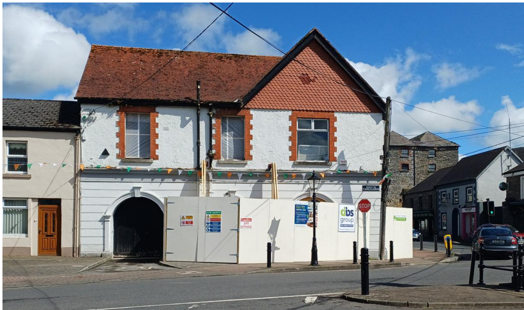
Figure 5: Fashion and Textile Design Hub (under construction) at former Bank of Ireland, Market Square
