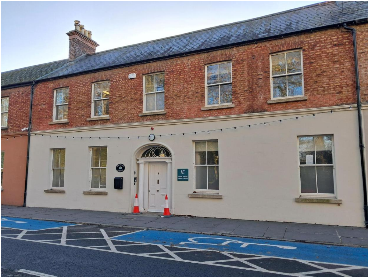
Figure 8: Monasterevin Daycare Centre and Health Centre
