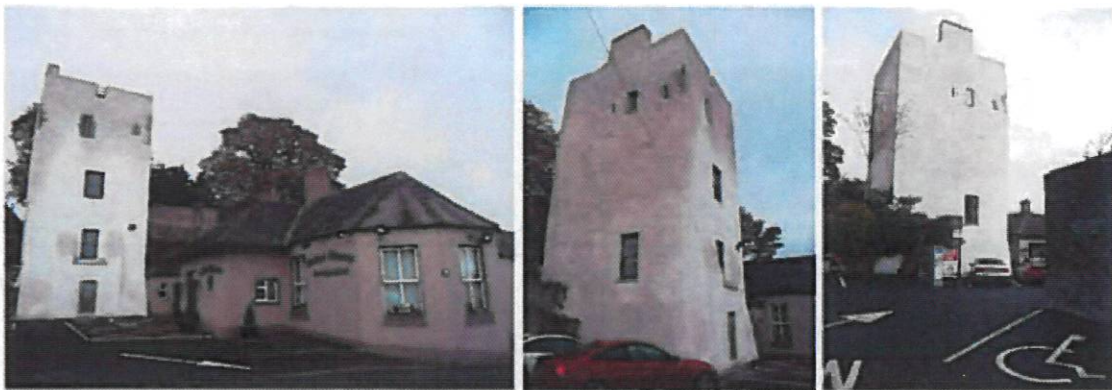
Harled rendered kildareGate house with base wall batter and Leinster Lodge
