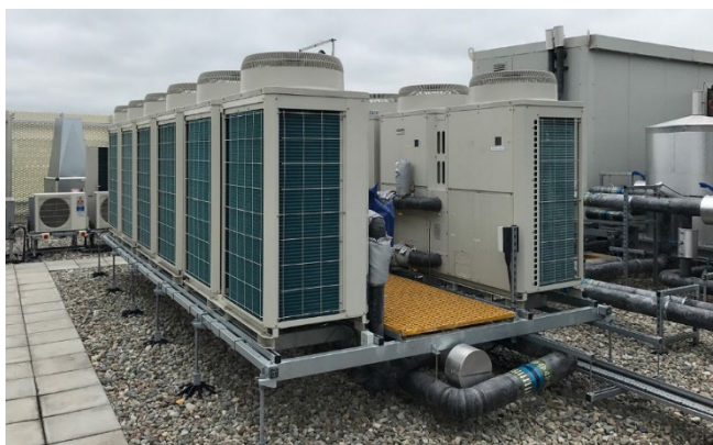
Figure 6.0 Commercial Air Source Heat Pump
