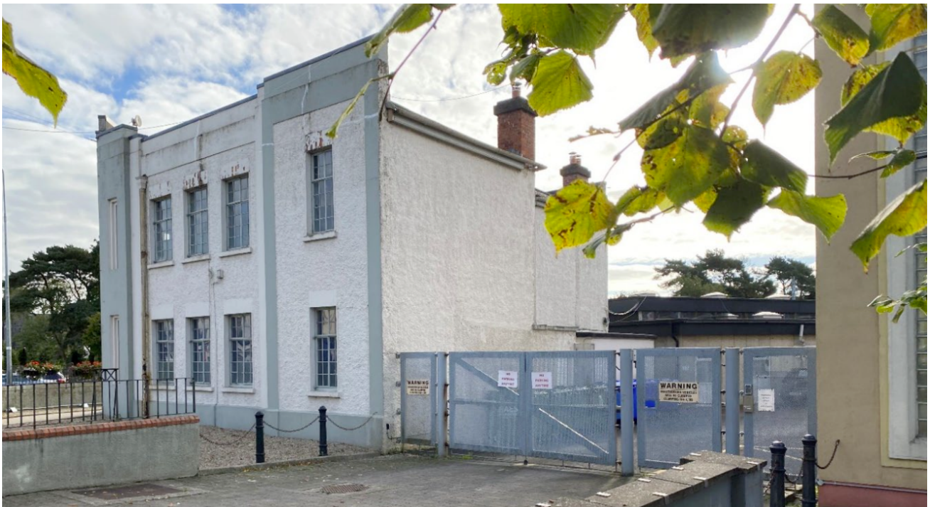
Figure 8: Google earth screen capture, existing County Library and shared entrance to yard beyond
