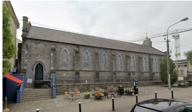
Figure 11: Google Street screen capture: Current Town Hall
