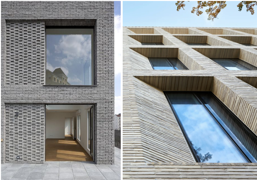
Fig. 23,24 Material Reference: brick window reveals
