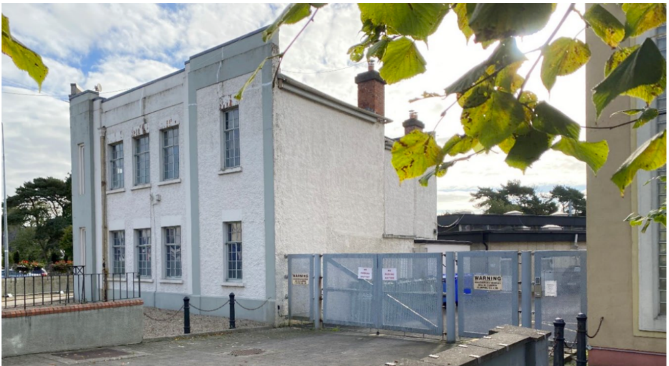
Fig. 2 Google earth screen capture, existing Liffey Terrace elevation
