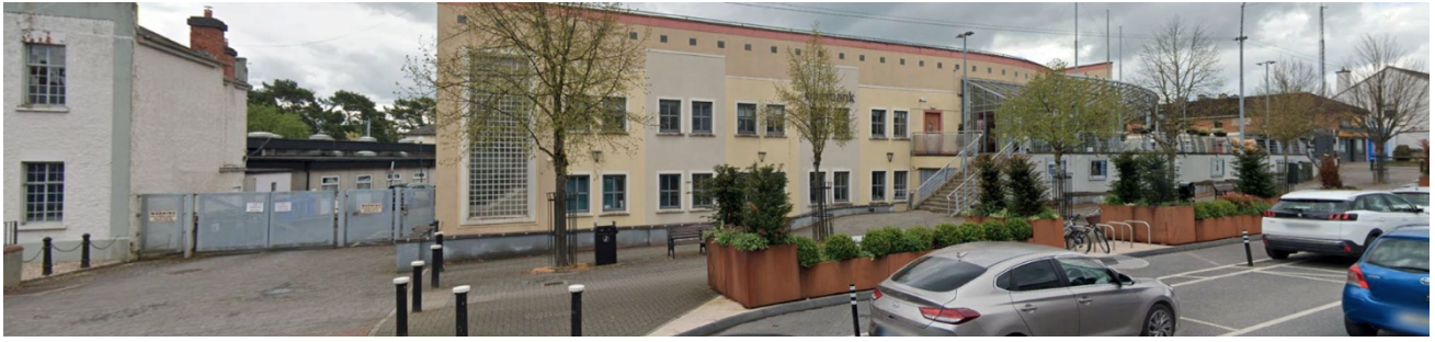
Fig. 3 Google earth screen capture, Shared rear access and Library HQ
