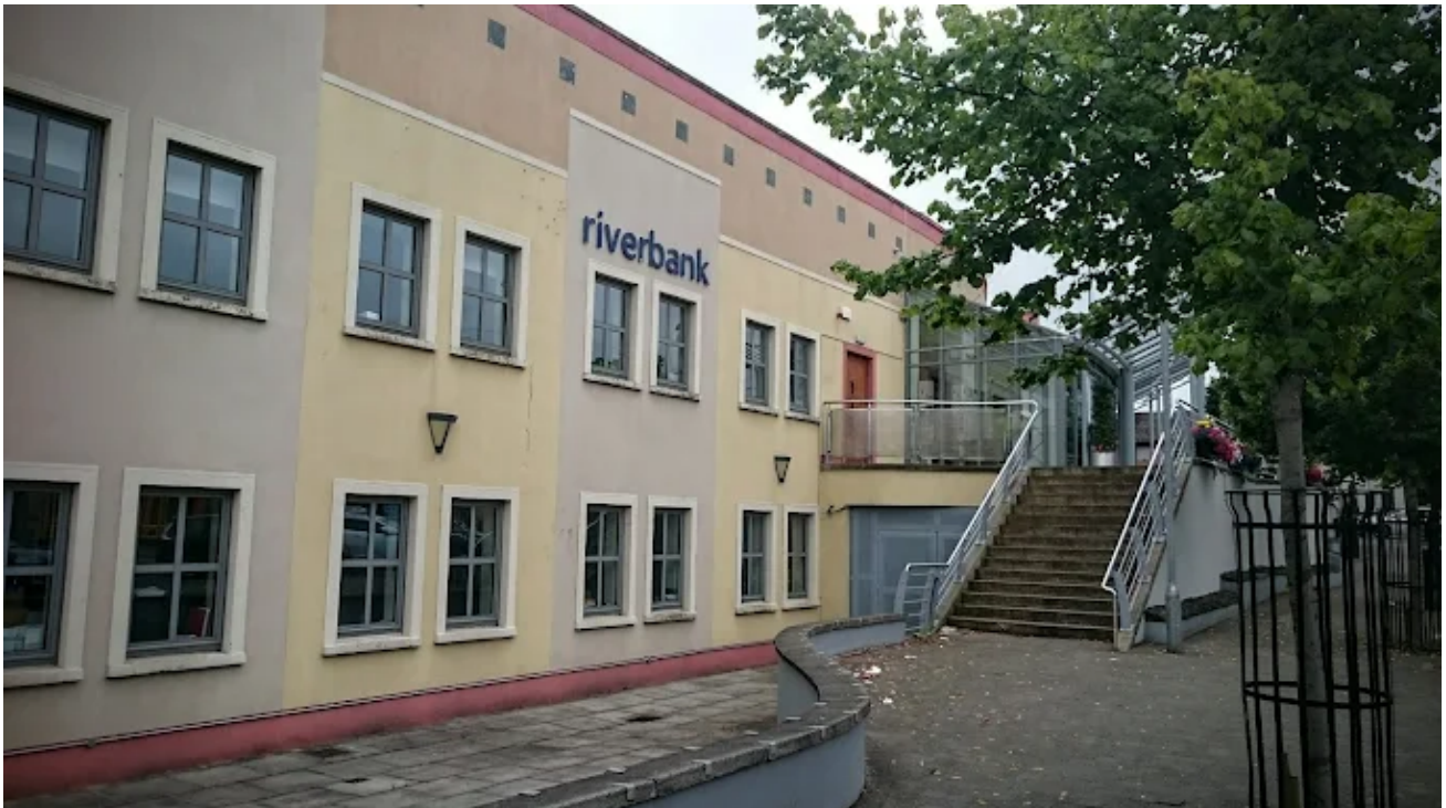
Fig. 11 Existing stepped entrance condition to Riverbank Arts Centre.
