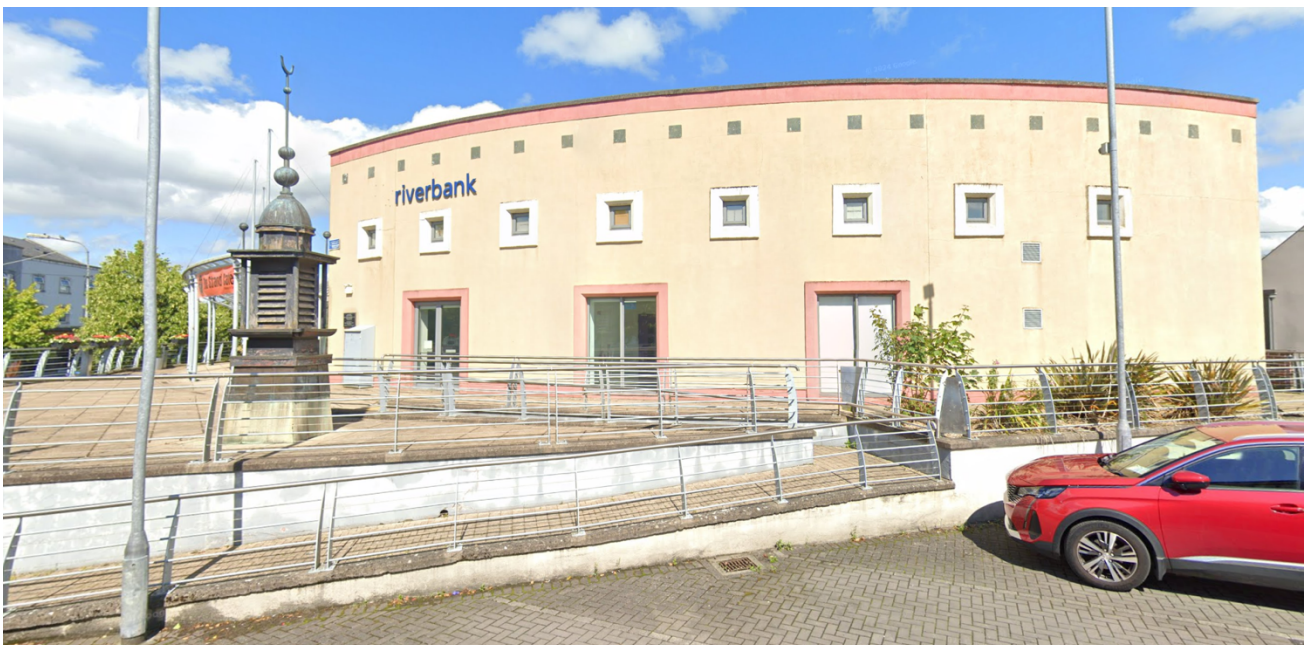
Fig. 5 Google earth screen capture, existing Liffey Terrace elevation
