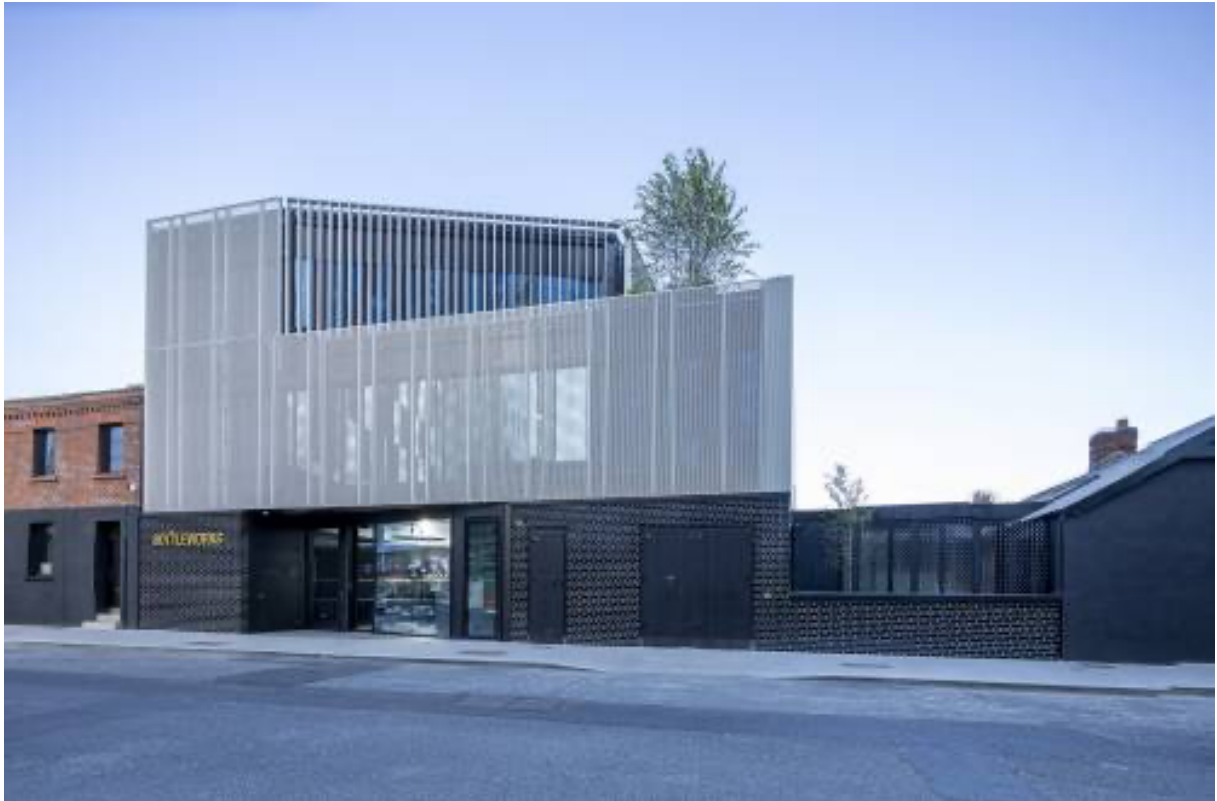
Fig. 21 Material Reference: Perforated metal at the Bottleworks, Barrow Street, Dublin, Henry J Lyons
