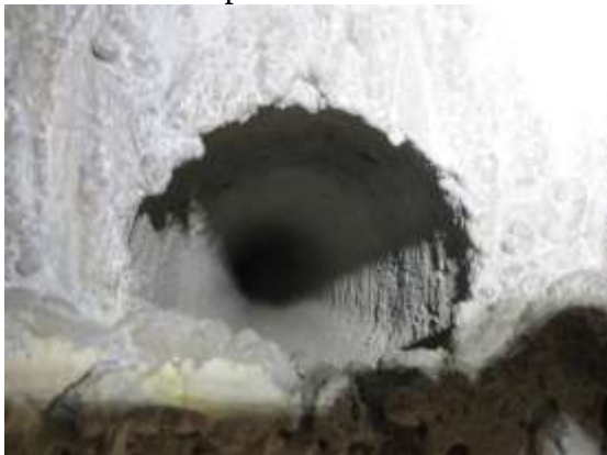
Plate 4 Hollow pre stressed concrete floor of roof void
