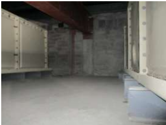
Plate 4 Hollow pre stressed concrete floor of roof void
