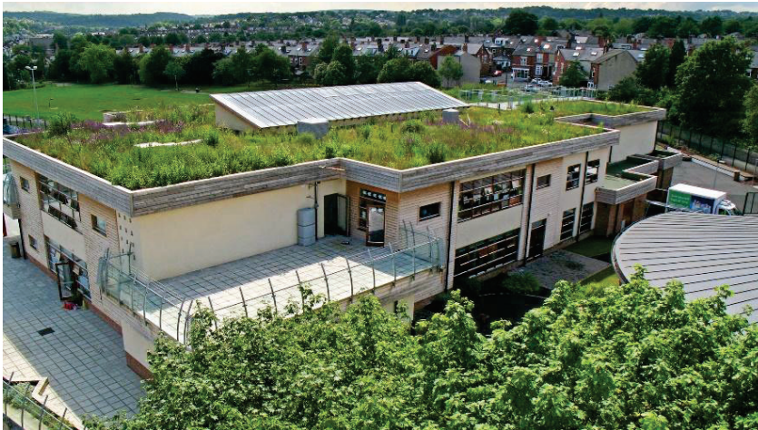
Figure 4-5 – Example Green Roof Build up on a school building (Source: CIRIA C753 Sharrow School green roof)
