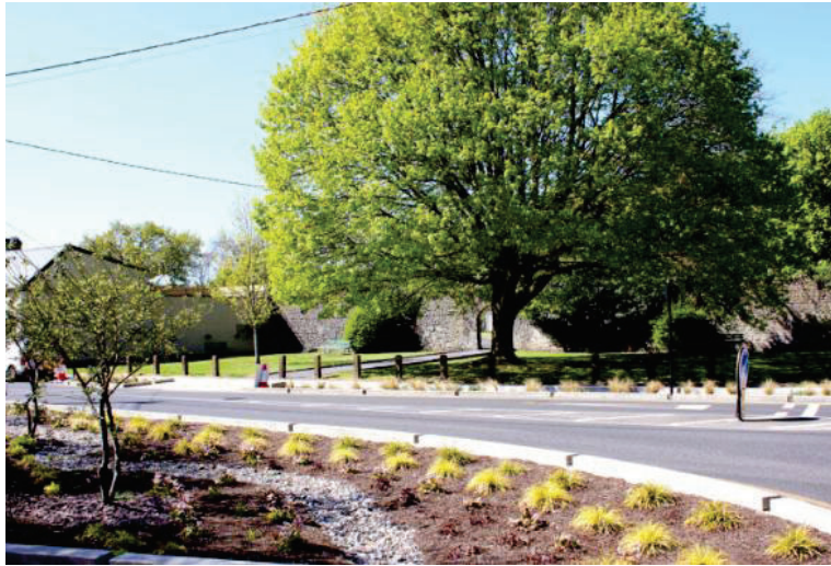
Figure 4-10 - Example of a raingarden adjacent to a roadway (Carlow Town)
