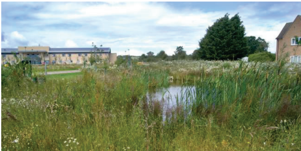
Figure 4-13 - Example of a Retention Pond (North Cotswold Hospital)
