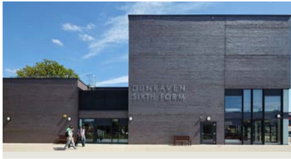
Figure 144: A robust, clearly defined secondary school building addresses the street through a strong frontage, active ground-floor entrances and large windows, creating a civic presence, natural surveillance and a welcoming interface with the public realm. Dunraven Sixthform, London © hamsonbarronsmith
