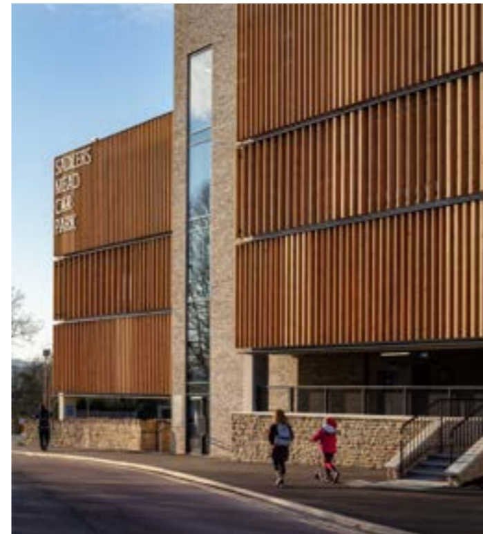
Figure 114: Building with timber-louvered facade. Sadlers Mead multi-storey car park. ©vincenttimber
