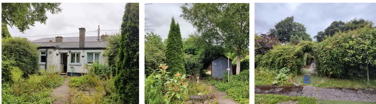
Above: Photographs showing the back of 13 Sallins Road taken in July 2024.
