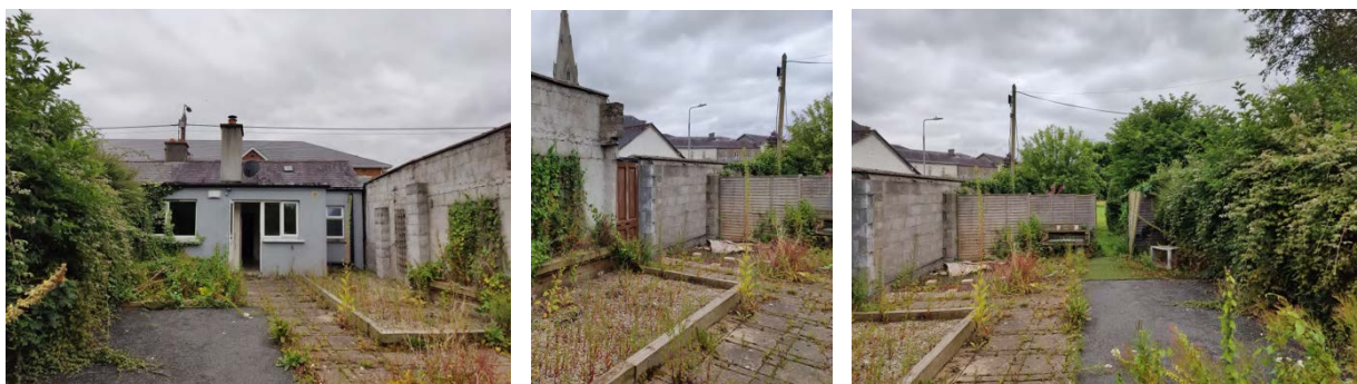
Above: Photographs showing the back of 18 Sallins Road taken in July 2024.
