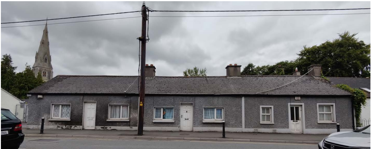
Above: Photographs showing the front of 13, 18 Sallins Road and Beaufort Cottage taken in July 2024.
