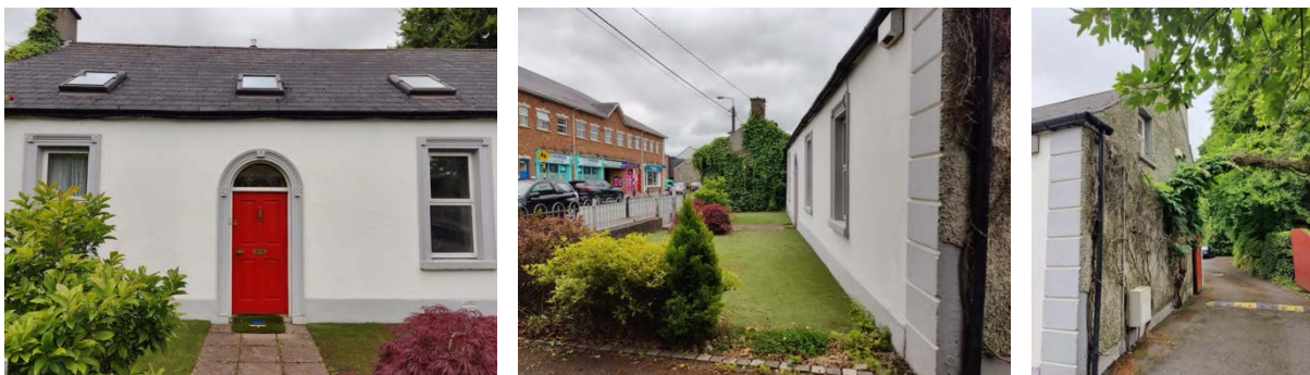
Above Left: Photograph showing the front door of Beaufort. Above Middle: View of the front garden. Above Right: View of the side elevation of Beaufort.
