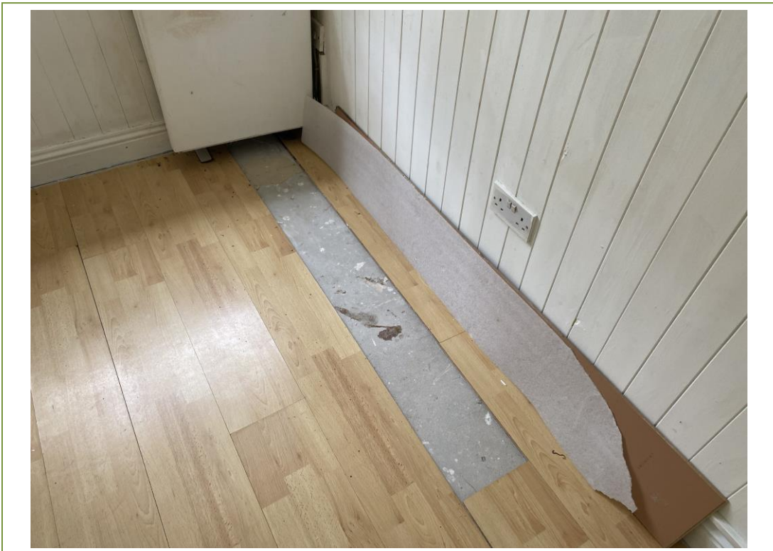
Bare concrete floors
