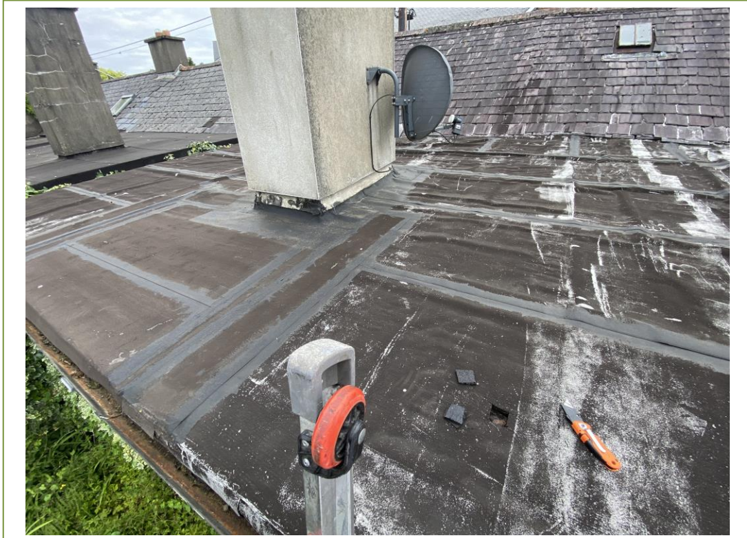
Felt sampled from the flat roof areas
