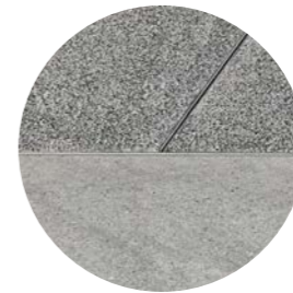
Exposed Aggregate Concrete
