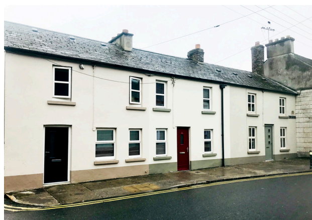
Figure 2.25: Refurbished houses on Offaly St. (July 2020)
