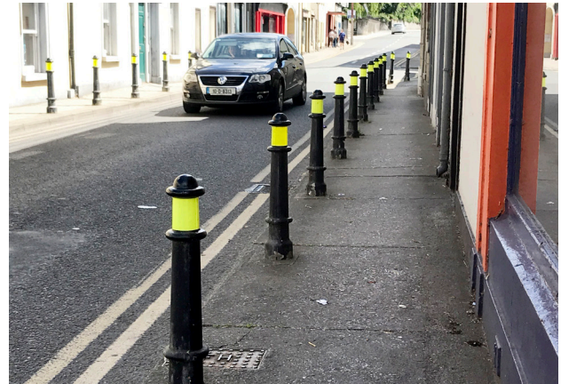
Figure 2.31: Excessive bollards on Offaly Row
