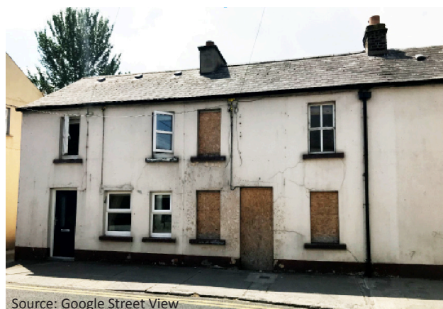
Figure 2.24: Derelict houses on Offaly St. (August 2018)
