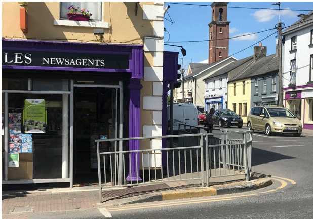
Figure 2.30: Non-pedestrian friendly railings at Emily Square
