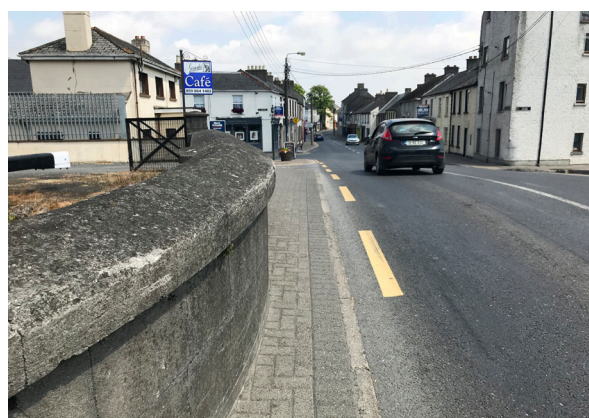
Figure 2.38: Substandard footpath on Augustus Bridge
