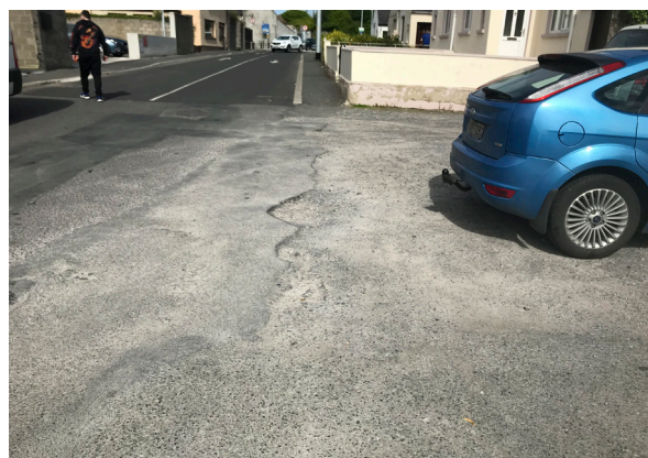
Figure 2.36: Lack of footpath on Meeting Lane
