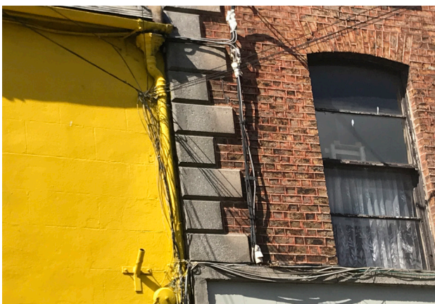
Figure 2.32: A proliferation of wiring on Leinster Street
