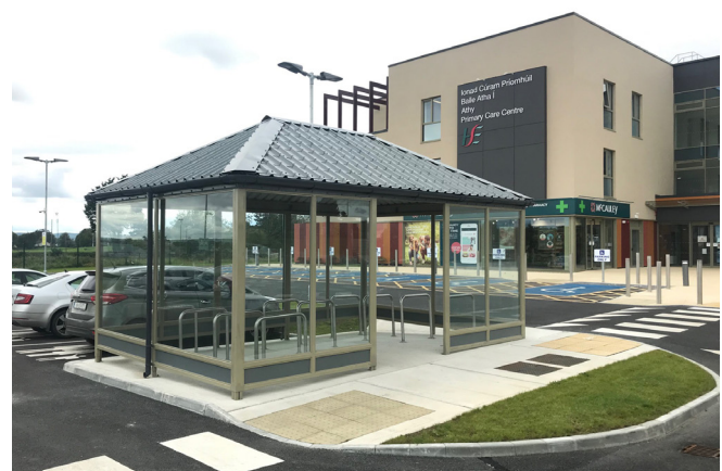
Figure 2.41: Cycling facilities at Athy Primary Care Centre
