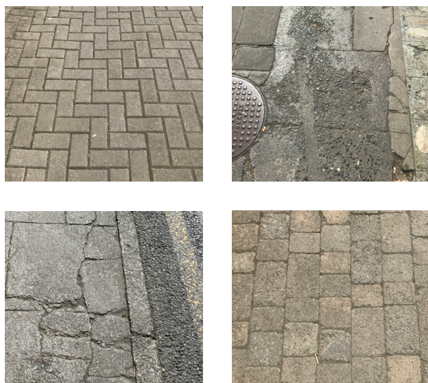
Figure 2.37: Varying pavement standards within town centre
