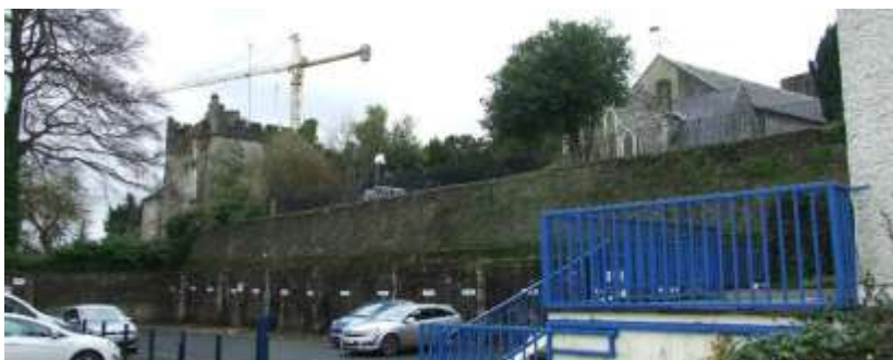
Fig.89: View of retaining wall, St David's Castle and COI from former rectory site
