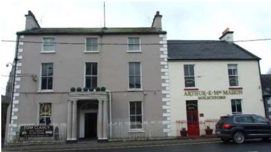
Fig.44: Former house beside Chapel Lane on the Dublin Road
