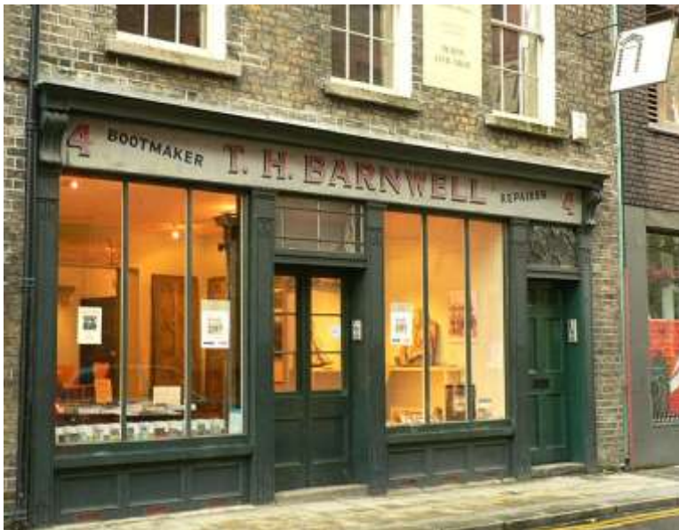
Fig.110: Shopfront refurbishment, Castle Street, Dublin (Dublin Civic Trust)
