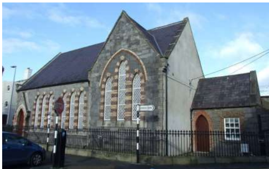
Fig.99: Stone façade with decorative brickwork
