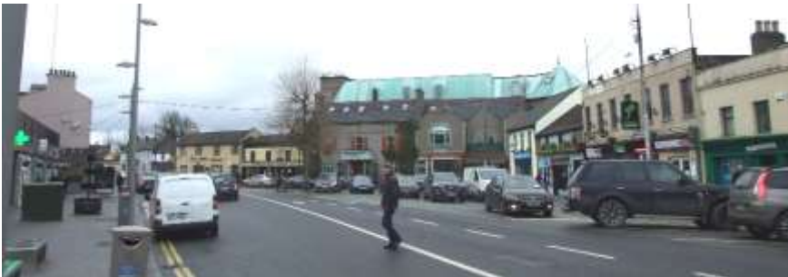
Fig.42: East and south sides of Poplar Square from North Main Street
