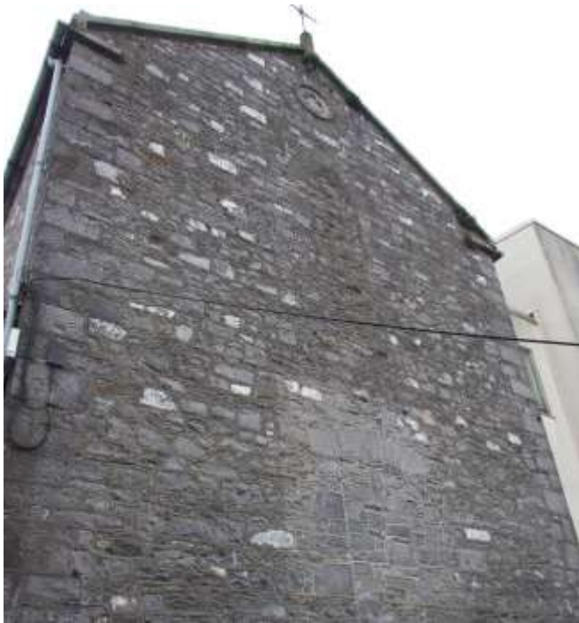
Fig.101: Exposed rubble stone wall
