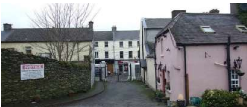
Fig.87: View of gate and approach to St David's COI towards North Main Street
