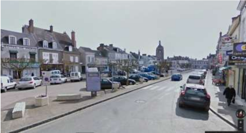
Fig.121: Neuville aux Bois, France. Google image of the main street, 2009 prior to refurbishment of the Main Street.
