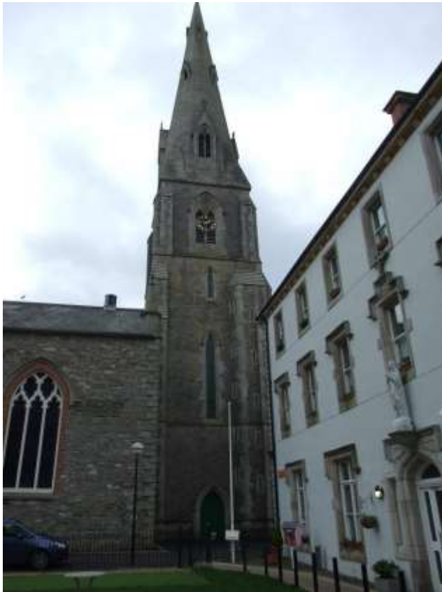
Fig. 27: RC Church of Our Lady and St David and convent building
