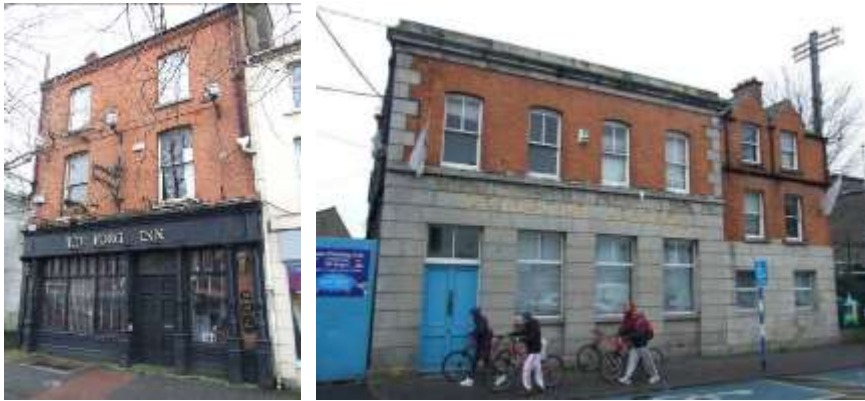
Fig.98: Use of brick in historic elevations
