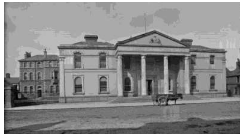
Fig. 10: Naas Courthouse (1805-10), Lawrence Collection, c. 1900
