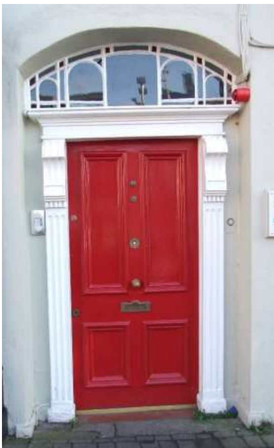
Fig.104: Decorative fanlight on South Main Street
