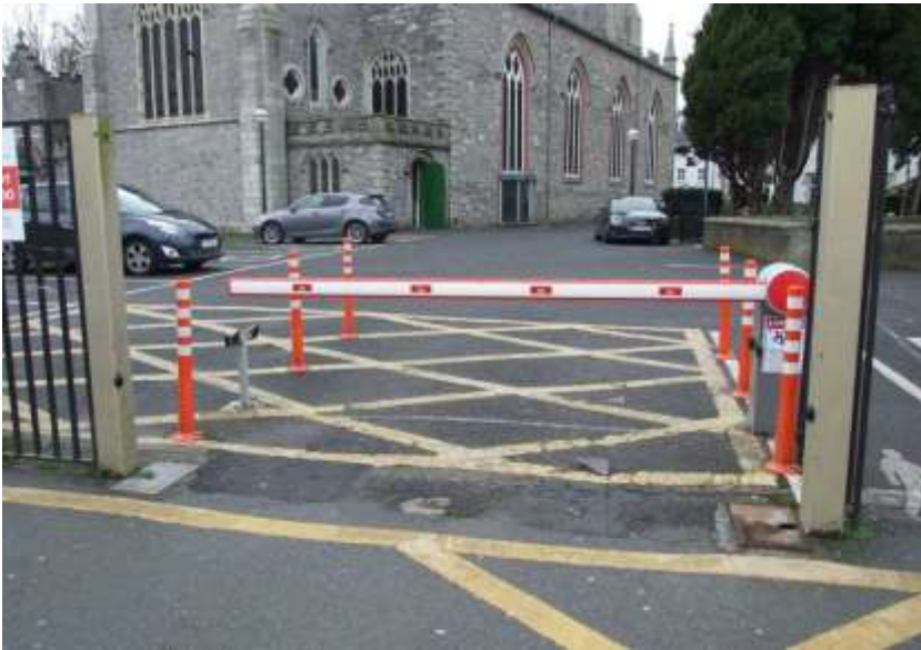
Fig.118: Visually intrusive access controls detract from the historic structure
