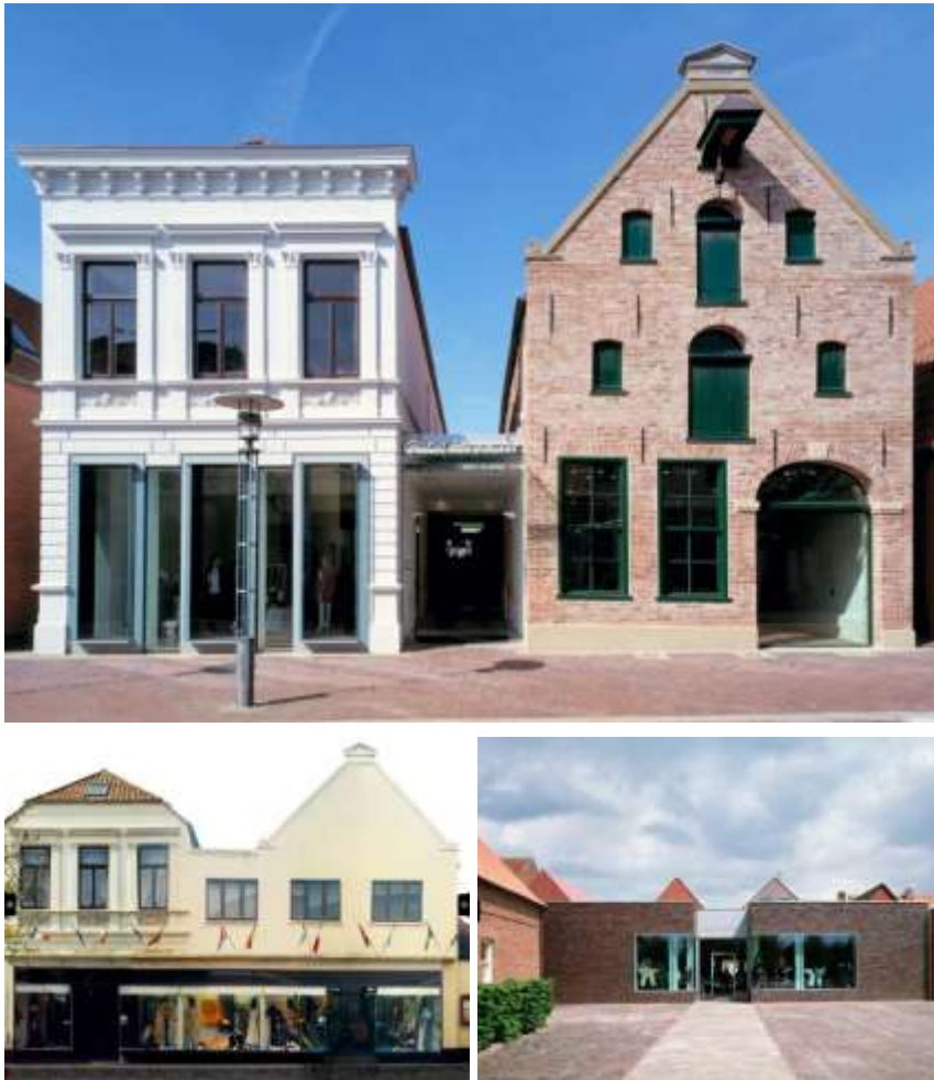
Fig.111: Street renovation, Norden, Germany by Riemann Conservation Architects. Two of some ten buildings refurbished. Historic fabric was revealed and reinstated. Note the contemporary addition to the rear of the site to allow for a new shopfront and access.
