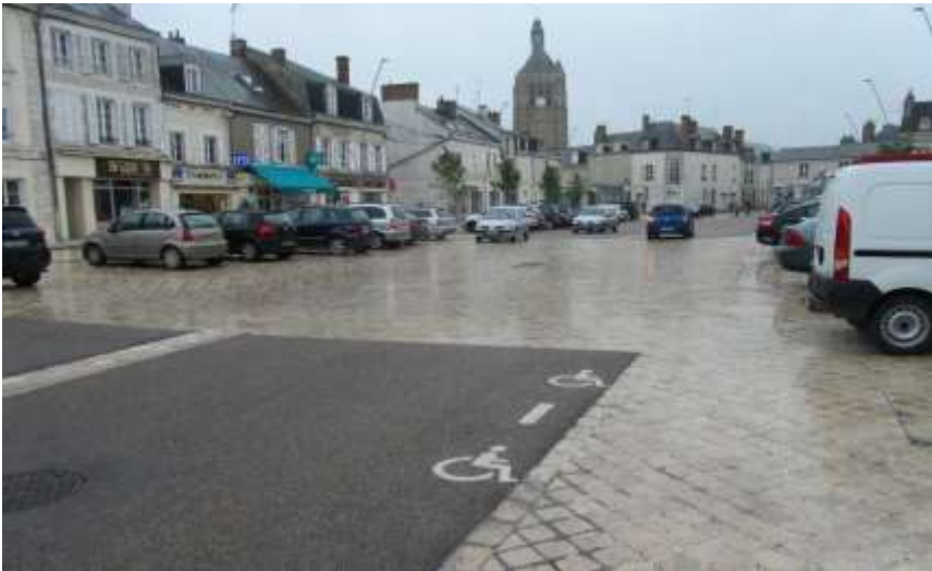
Fig.122: Neuville aux Bois, France, following refurbishment of the main street. Note the continuation of stone used for paths into areas for parking and part of the public street to give the appearance of a square and diminish the character of a 'road'. Note also that all kerbing and most signage has been removed.
