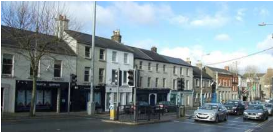
Fig. 25: West side of South Main Street
