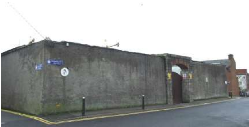
Fig.78: Boundary of Market to rear of Town Hall
