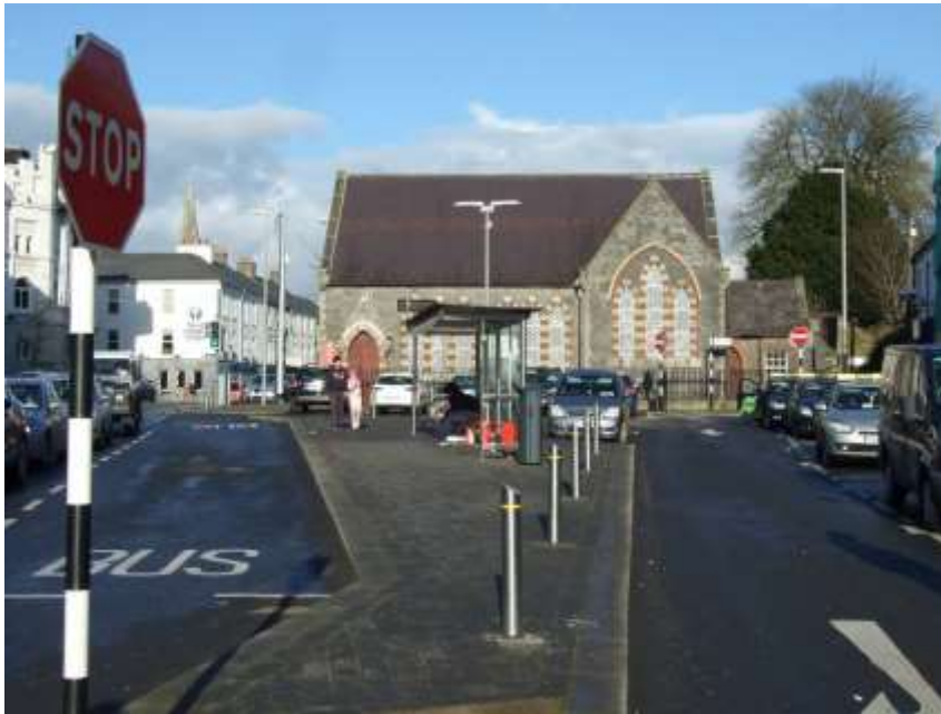
Fig. 120: Proliferation of kerbs and separate road surfaces for parking and access, signage, lighting masts, bins and a bus stop have a negative impact on the most important historic public space in the town
