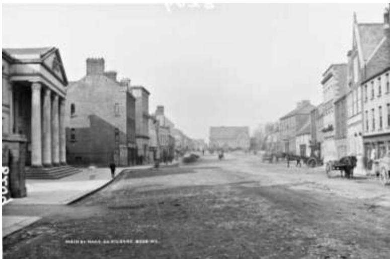
Fig. 17: South Main Street, Lawrence Collection, c. 1900
