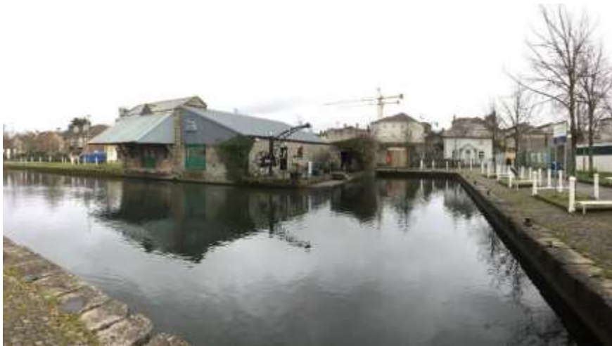
Fig.68: Canal Harbour Basin with historic warehouse structure
