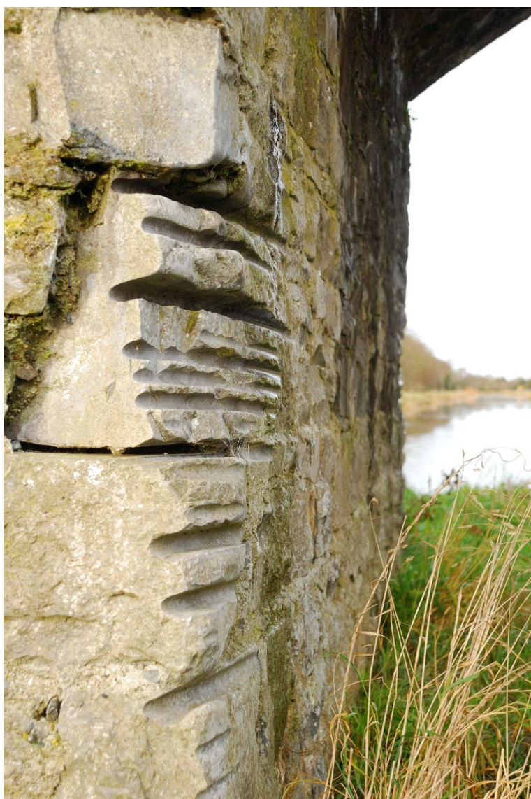
Rope wear marks from horse-drawn barges, Grand Canal
