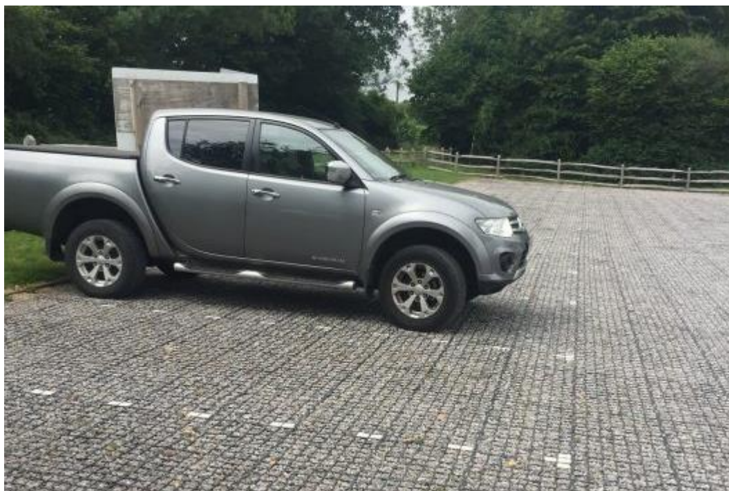
Fig 7 - "Geogrid" Geosynthetic Grass Reinforcing Grid (prior to Grass growth).
